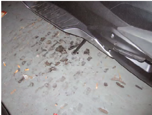
A surface dressing with many damage marks.
