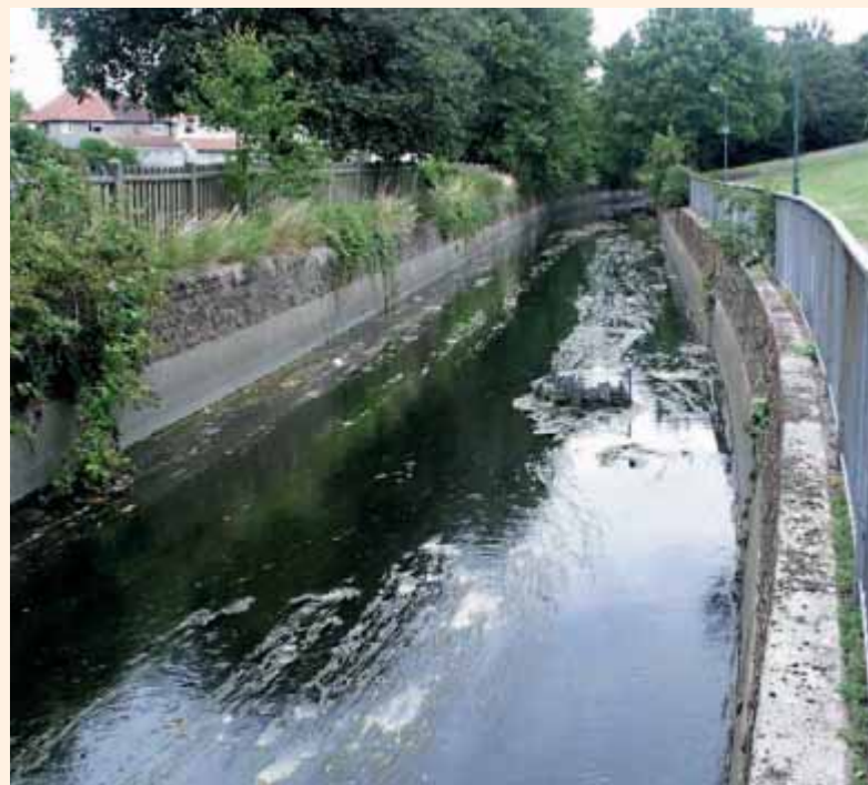
The river in 1999, before work began
