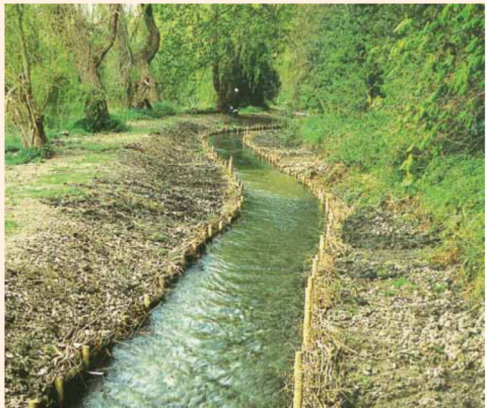
River channel narrowed using faggots (post-project, 1994)
