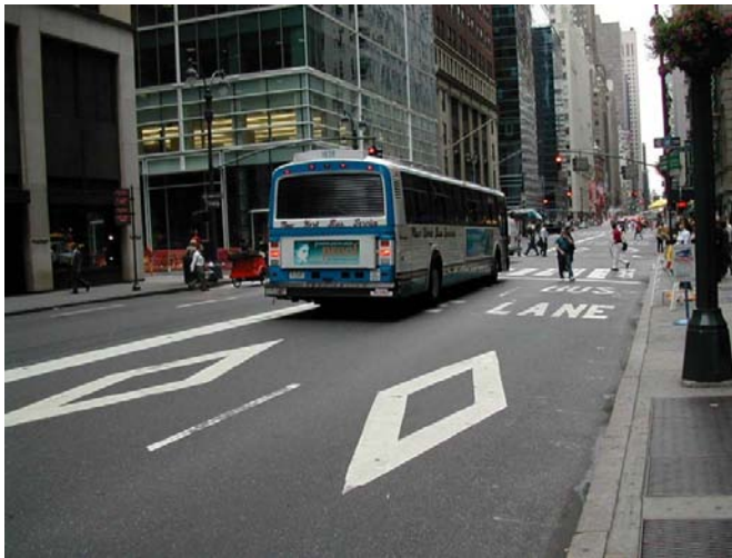
SOURCE: Kittelson & Associates, Inc. EXHIBIT 4-8 Dual Curb Bus Lanes (New York City)
