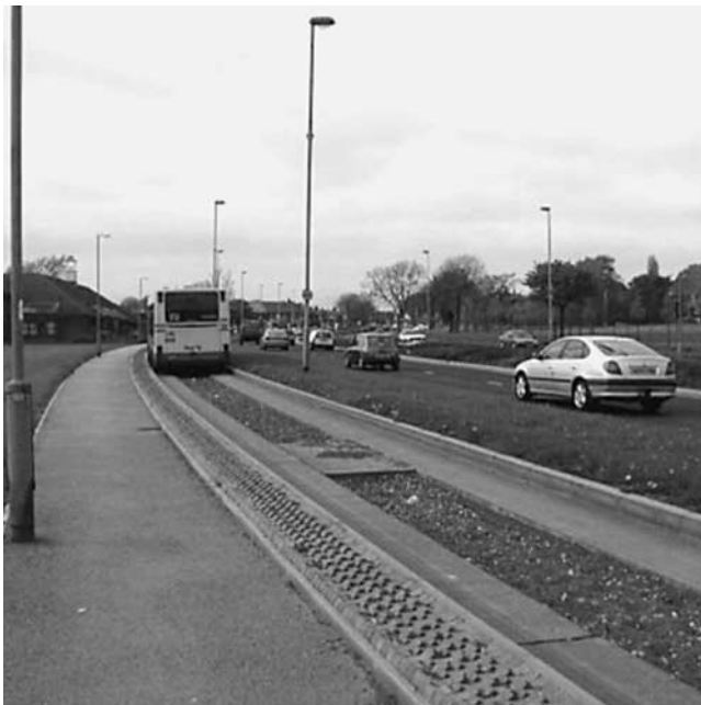
Photo 7-H. BRT guideway, Leeds.
