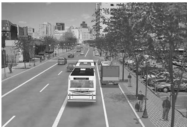
Photo 3-B. Interior bus lane, Silver Line, Boston.
