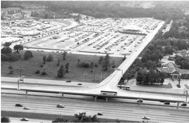
Photo 3-H. “T” ramp in Houston.
