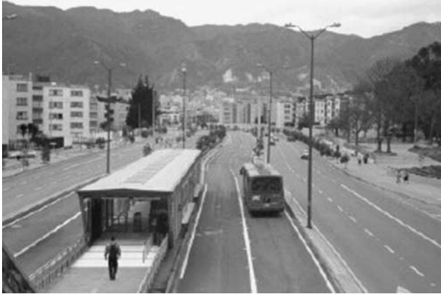
Photo 3-C. Median arterial busway, Bogotá.
