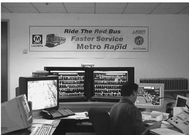
Photo 7-E. Central control room, Metro Rapid, Los Angeles.
