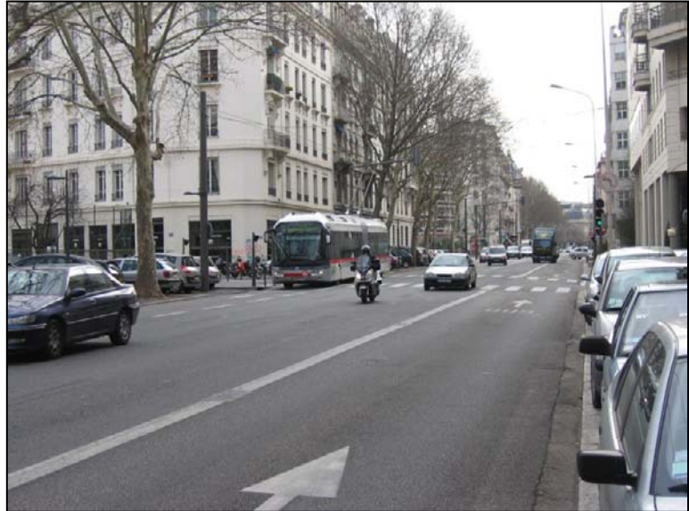
Photo 12: on Line C1 in Lyon, the decision to install unprotected side lanes can be a source of disruption for bus traffic (double-parked cars, delays or disruption due to kerbside parking, etc.) (source: Certu)
