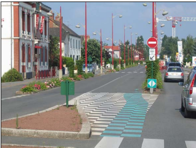
Photo 11: the installation of axial dedicated lanes in Rennes limits the effects of external disruption and makes the roadspace easier to understand as a whole (source: Certu)
