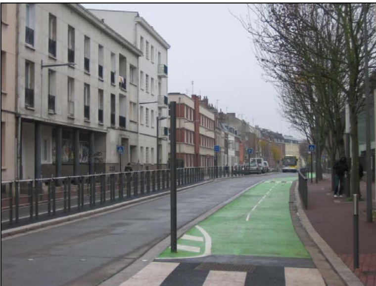
Photo 14: separate running in each direction for Douai's BHLS system, Évéole (source: Certu)
