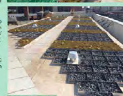
South Rooftop Complete
