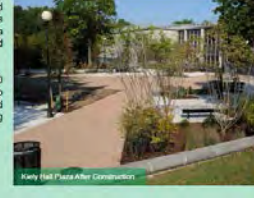
Kiely Hall Plaza After Construction
