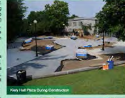
Kiely Hall Plaza During Construction
