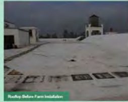
Rooftop Before Farm Installation
