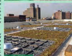
South Rooftop Complete
