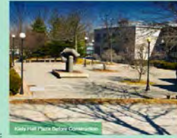
Kiely Hall Plaza Before Construction
