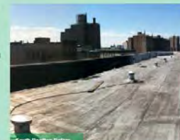
South Rooftop Before
