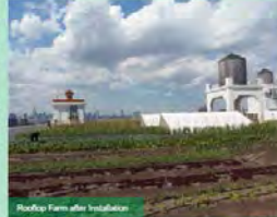
Rooftop Farm after Installation
