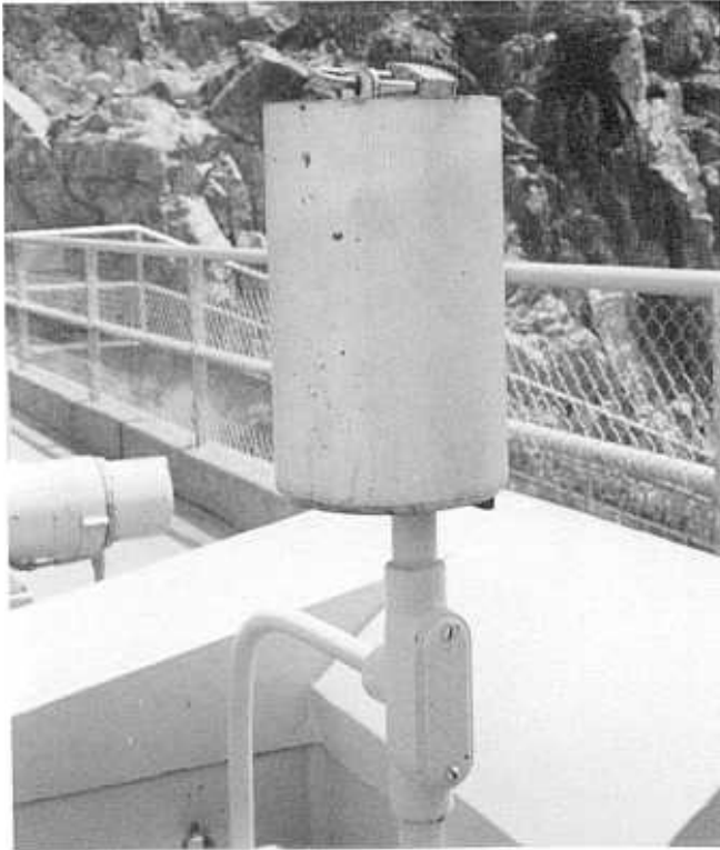
Figure 10-10.—Canister locked over assembly.
