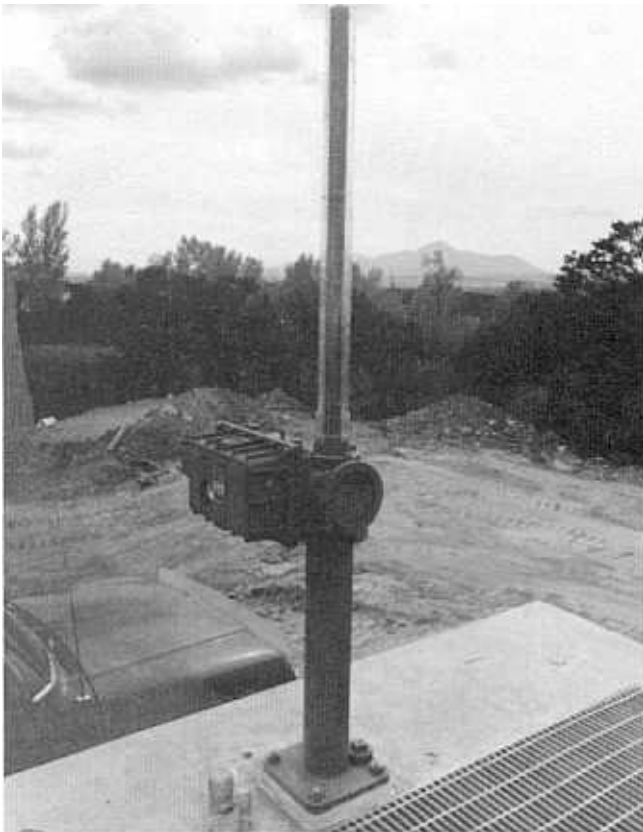
Figure 9-11.—Slide gate hoist.
