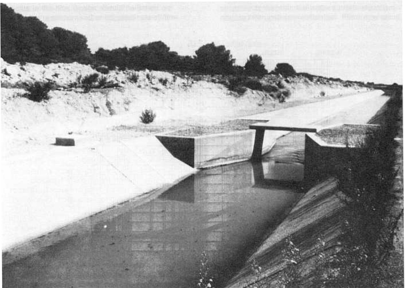
Figure 9-7.—Parshall flume.
