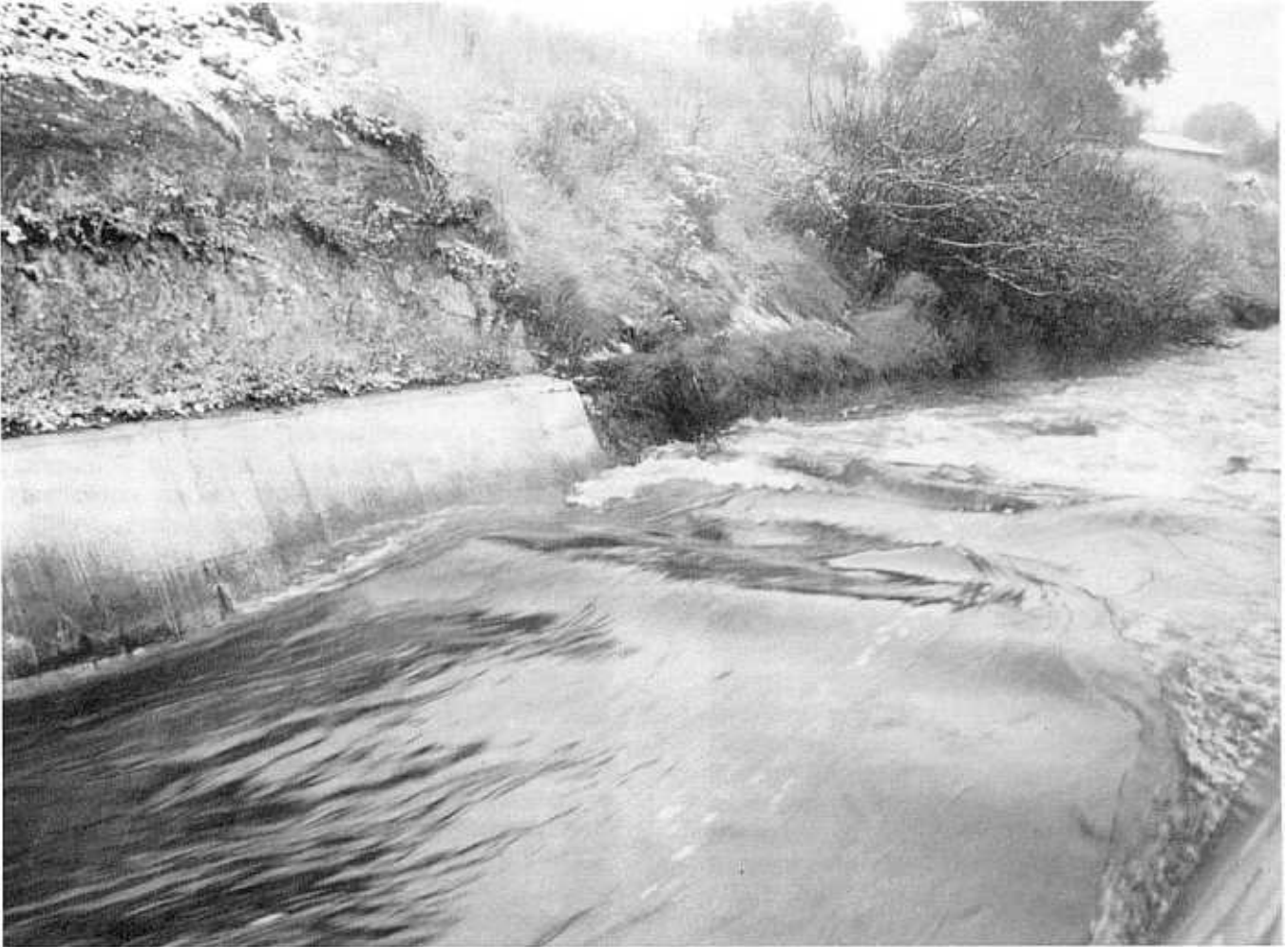
Figure 9-8(a).—Ramp flume.
