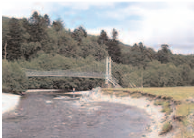
Figure 9: Bridge structure at risk of failing due to inappropriate location on an active river
