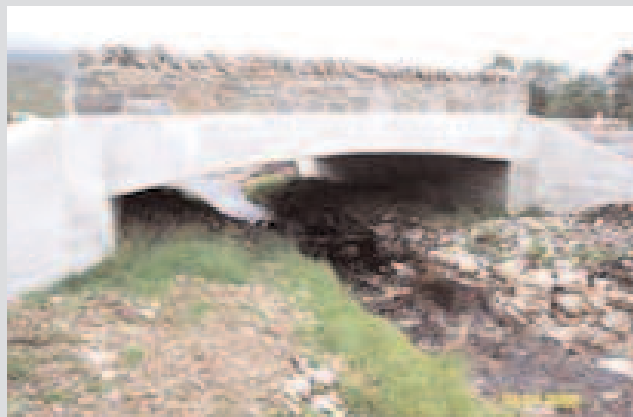
Figure 21 Bridge showing set back abutments (photo courtesy of Highland Council)
