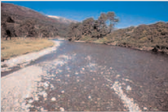
Figure 27 Ford crossing showing over-widened river and lower water depth
