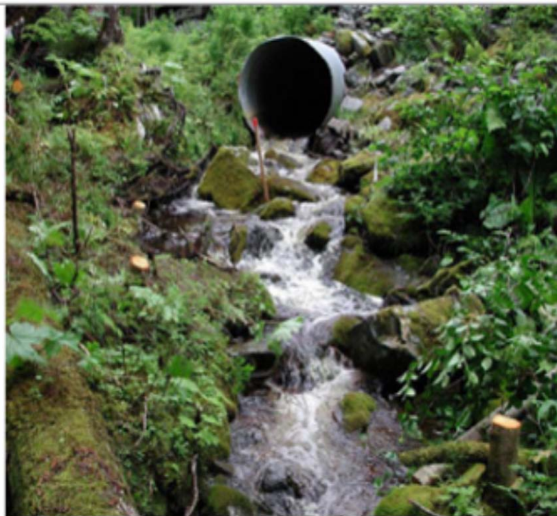
Figure I.1. Tributary to Bear Creek Culvert Outlet.
