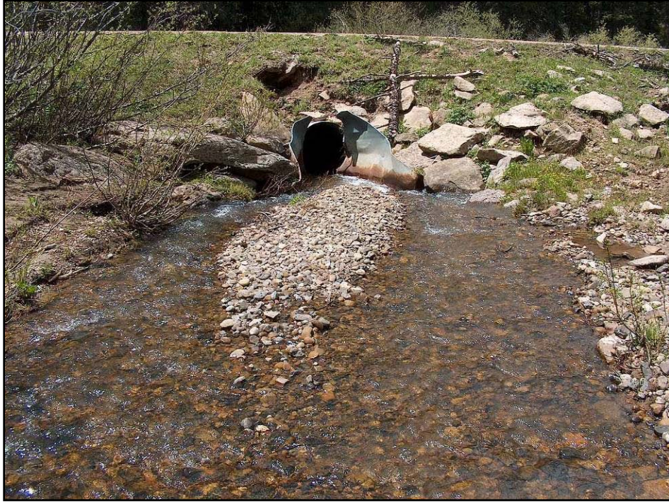
Figure H.2a. North Thompson Creek Culvert Inlet.
