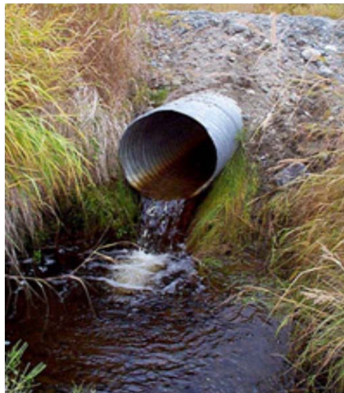
Figure 2.2. Perched Outlet, Leap Barrier.
