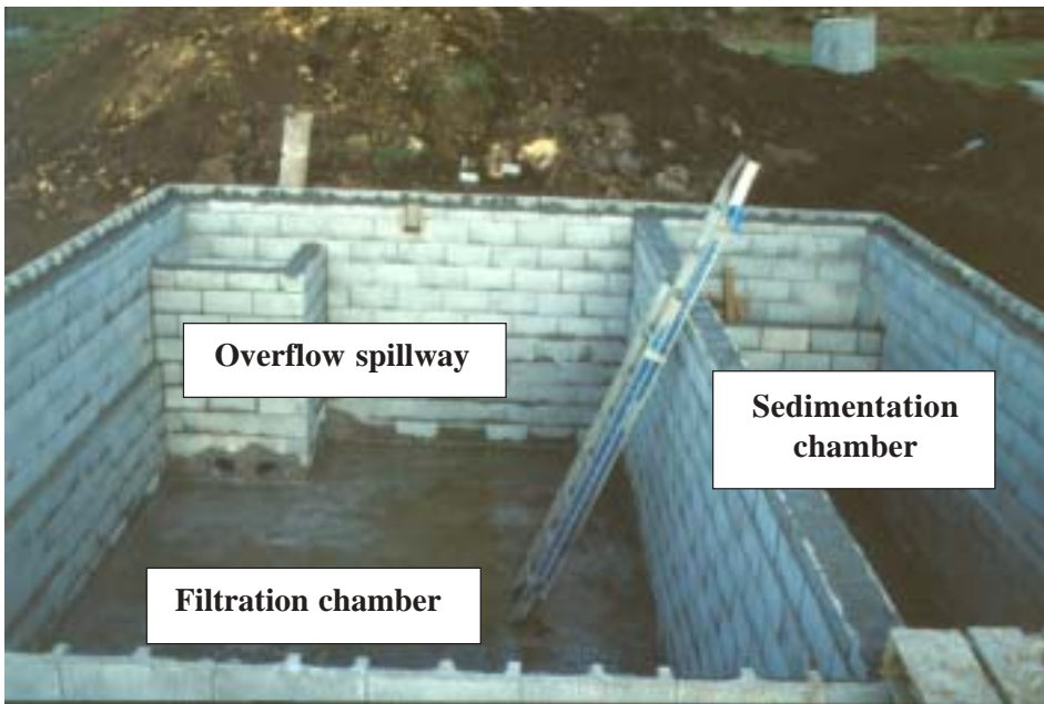
Plate 7-1: Unitec sand filter under construction showing various components
