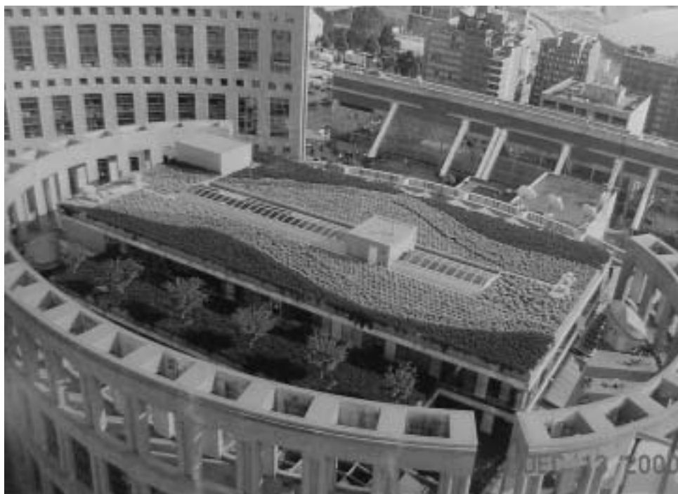
Plate 12-5: Greenroof as an aesthetic feature
