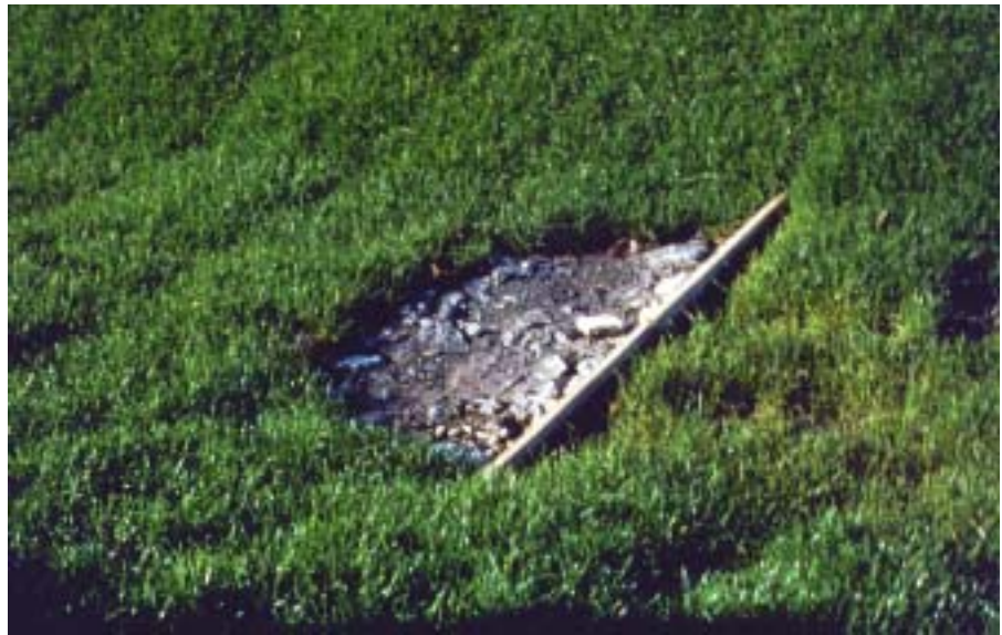
Plate 9-3: Detail of a swale check dam
