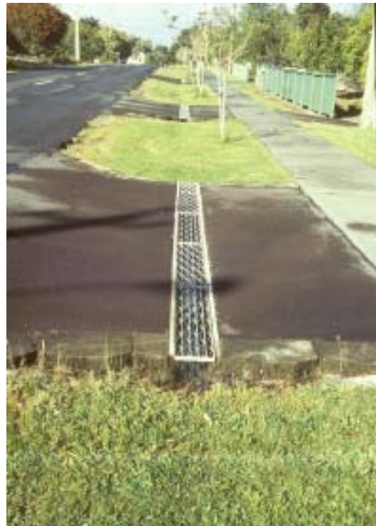
Plate 9-1: Example of a well designed and maintained swale
