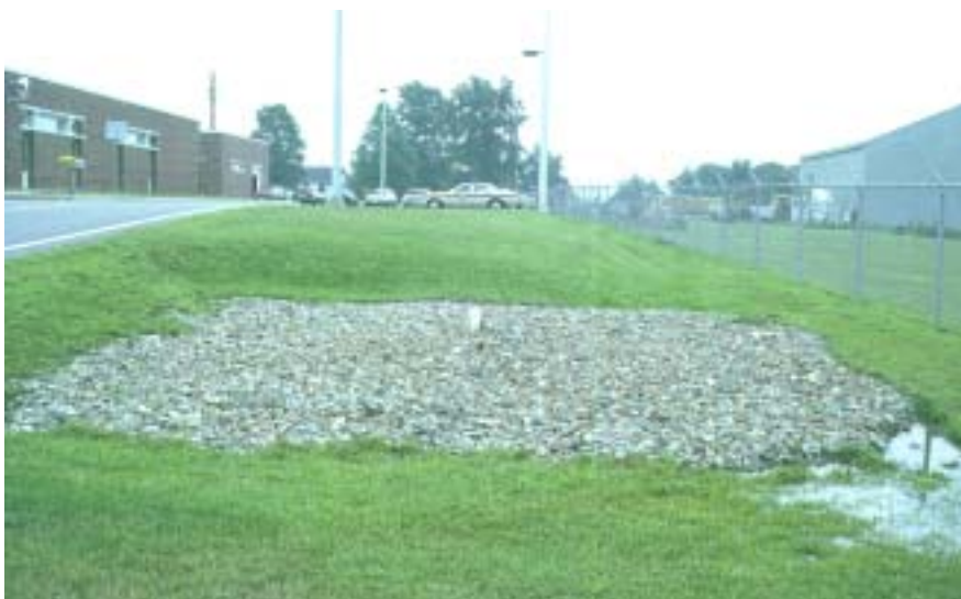
Plate 8-2: Infiltration trench with a swale for pretreatment
