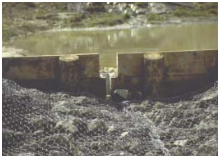
Plate 5-3: Outlet Structure Showing Multiple Storm
