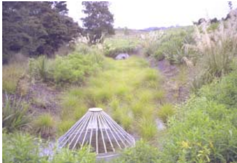
Plate 6-1: Small Well Landscaped Constructed Wetland
