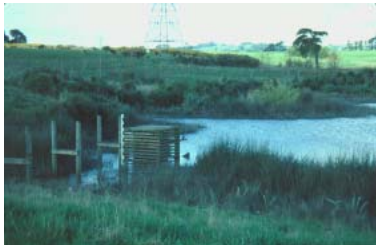
Plate 6-2: Larger wetland providing stormwater and wildlife benefits
