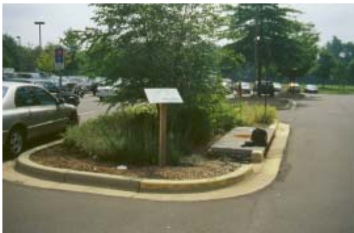
Plate 14-6: Well landscaped rain gardens in a commercial parking area
