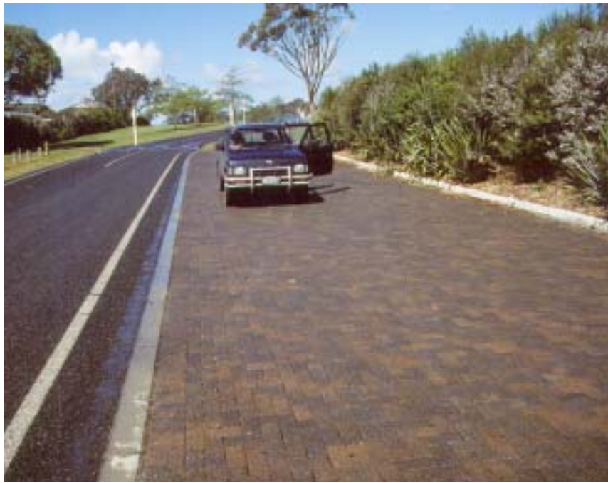
Plate 8-6: Example of a porous block parking area
