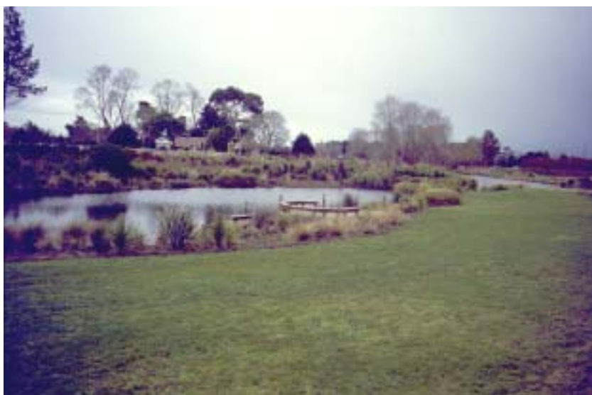
Plate 14-3: A well landscaped stormwater management pond
