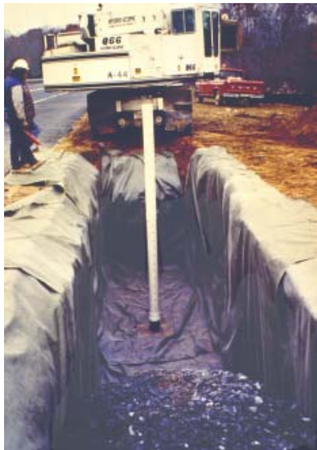
Plate 8-3: Infiltration trench under construction showing observation well, footplate, and fabric
