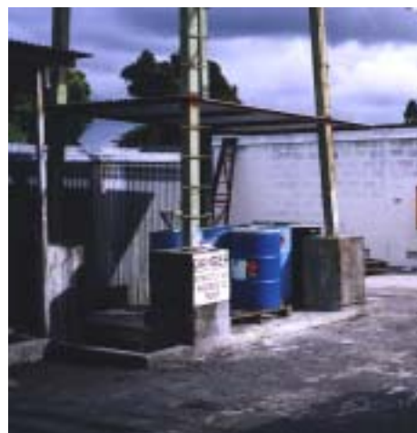
Plate 3-1: Chemical roof and bunding
