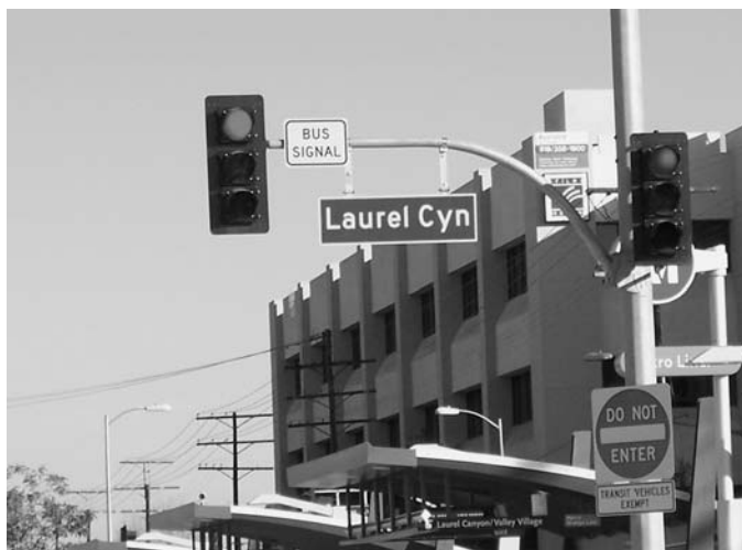
Figure 5-5. Bus signal sign mounted next to bus signal at intersection of Orange Line busway, Los Angeles.
