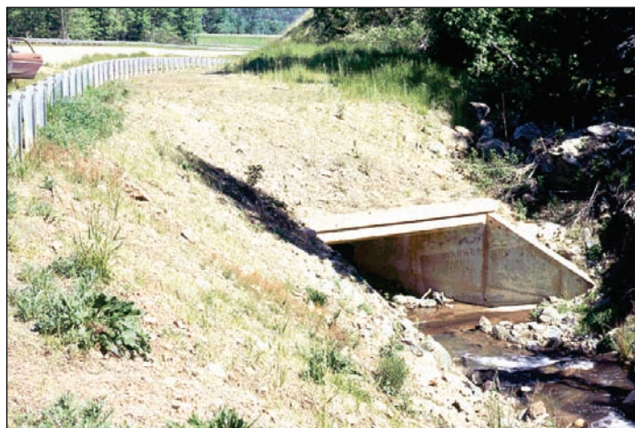
Figure 5.16. Fill warped to avoid inlet skew.
