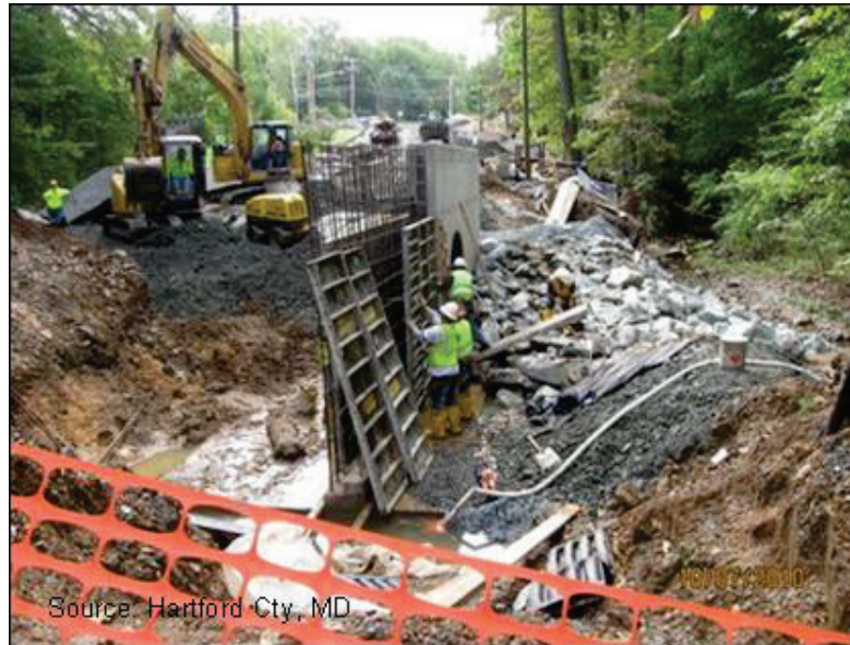
Figure 6.19. Concrete headwall and wingwall installation on pipe culvert.
