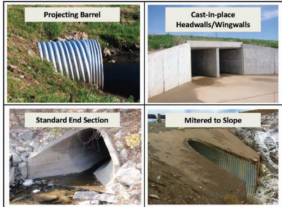
Figure 1.8. Four standard inlet types.
