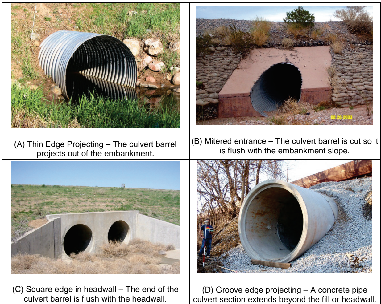
Figure 3.2. Typical inlet configurations.
