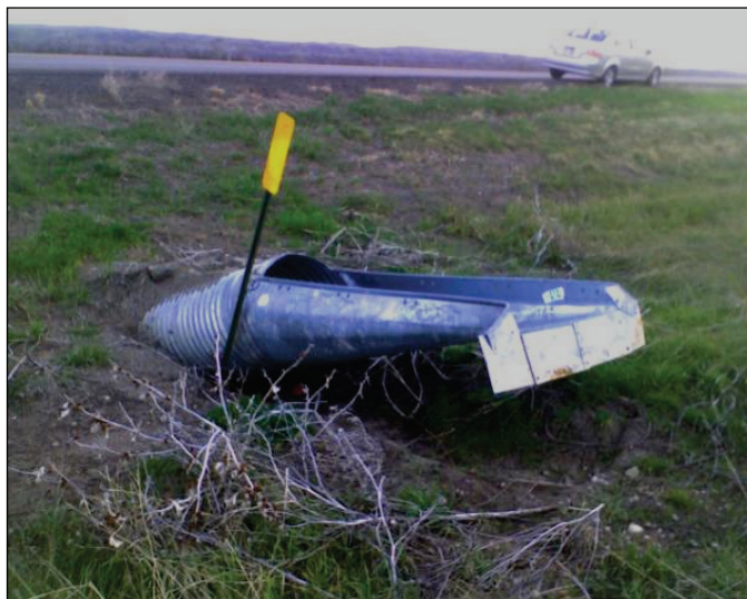
Figure 6.5. Buoyancy uplift.
