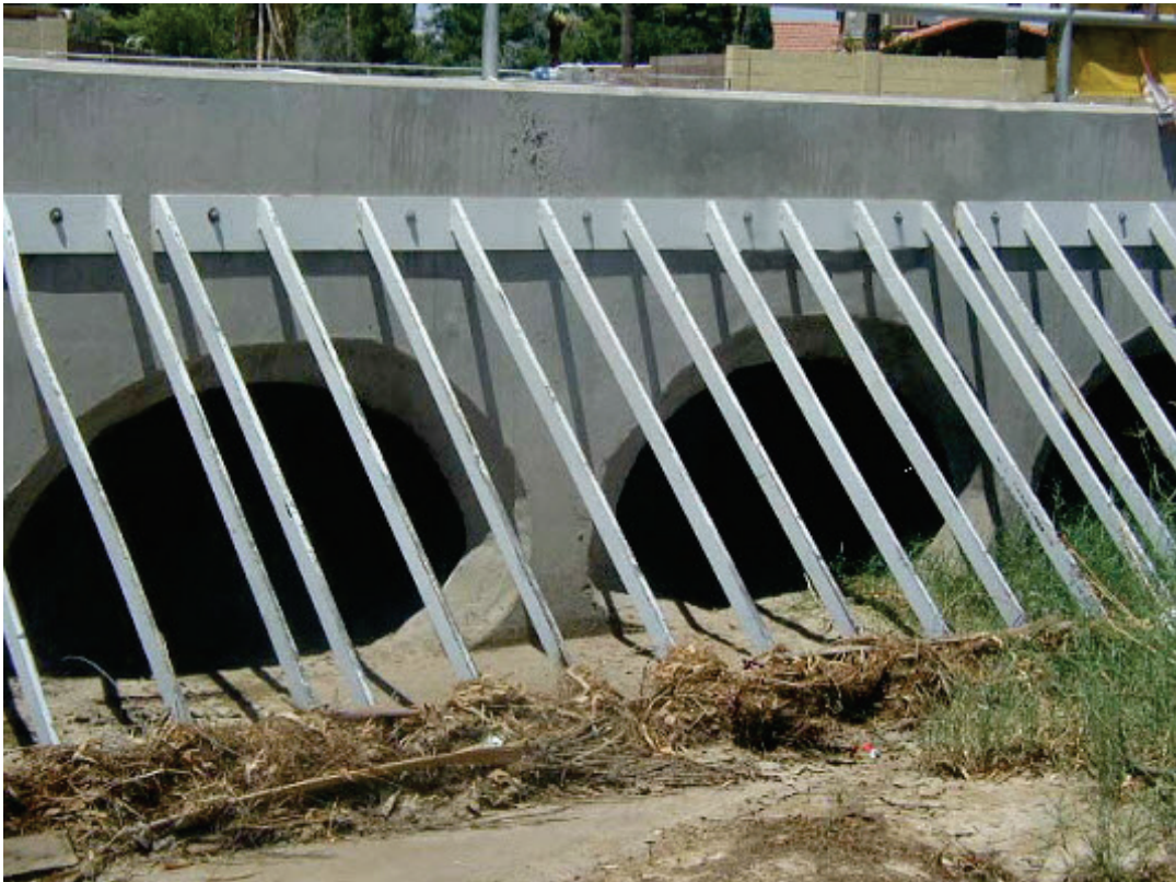
Figure 2.7. Steel debris rack in urban area.
