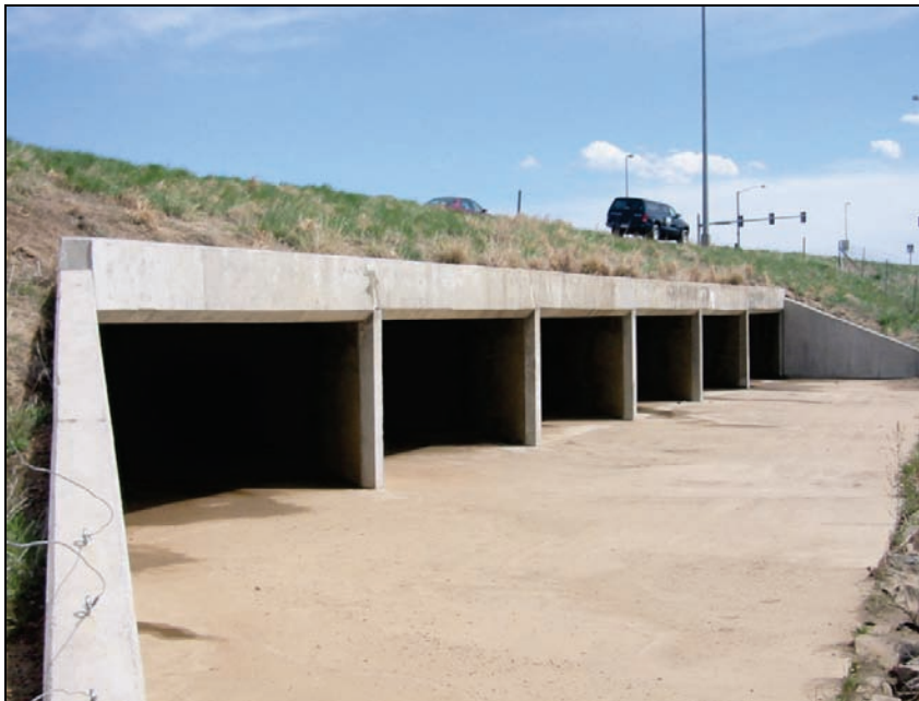
Figure 1.21. Multi-cell box culvert.
