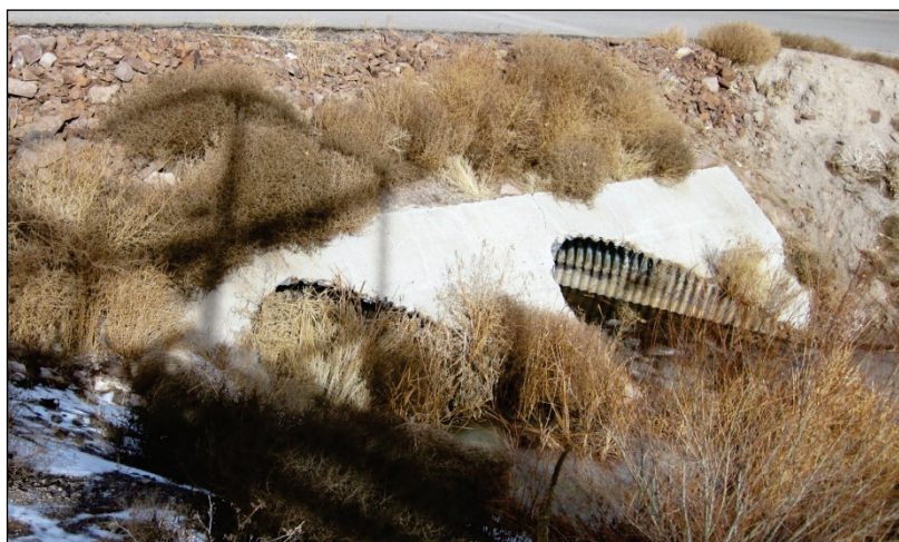
Figure 5.20. Slope paving around a mitered inlet.
