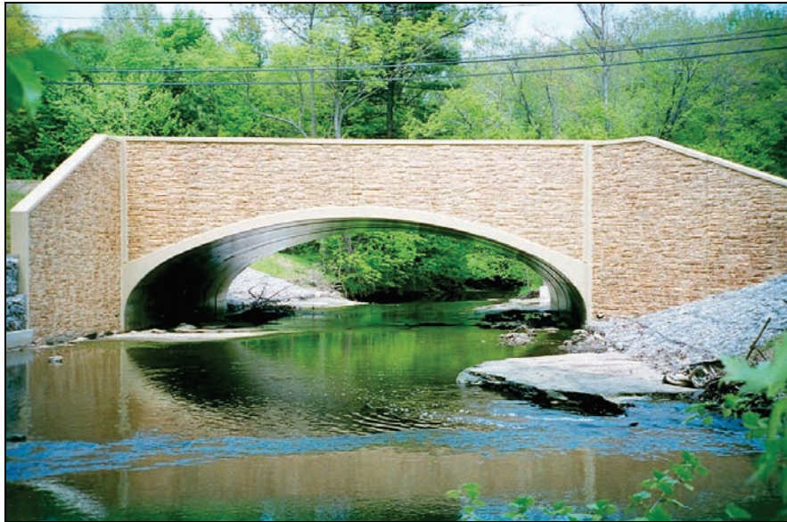
Figure 1.15. Long span culvert.
