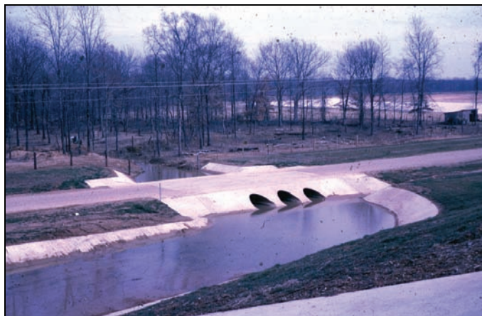
Figure 1.14. Vented low-water crossing.
