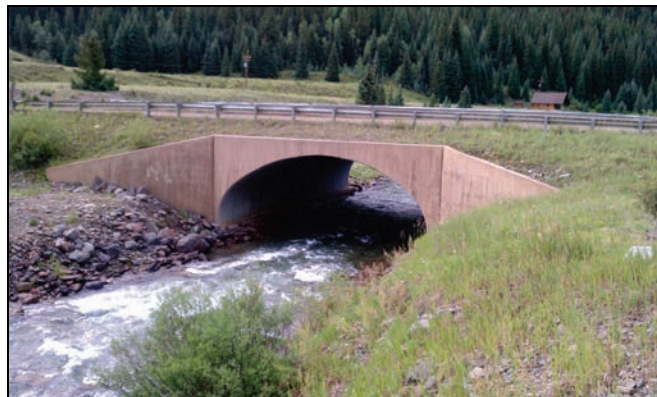
Figure 1.11. Open-bottom culvert.
