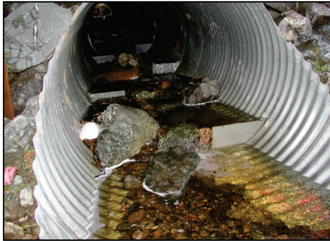
Figure 5.6. Alternating baffles.
