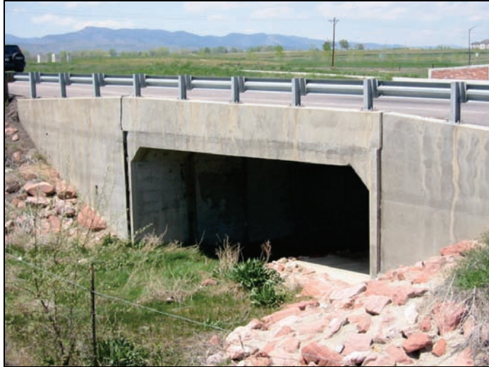
Figure 1.6. Concrete box culvert.
