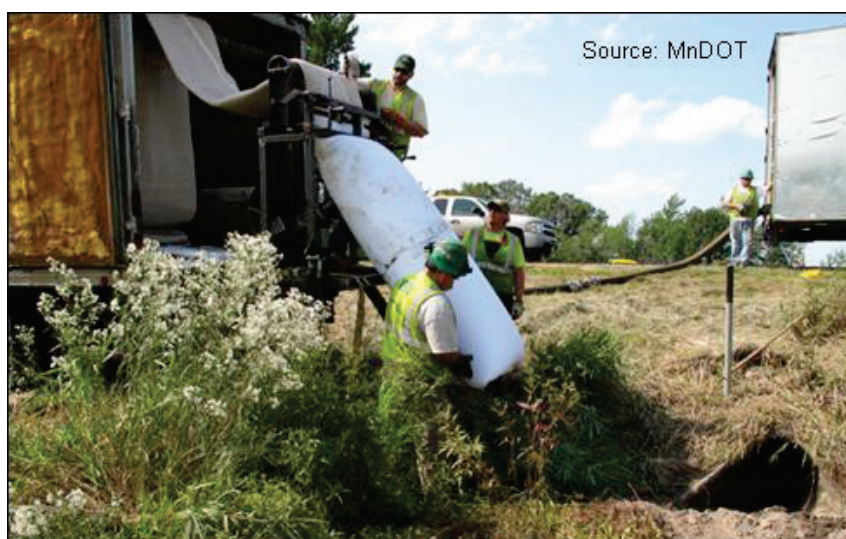
Figure 6.14. Cured-in-place liner installation.
