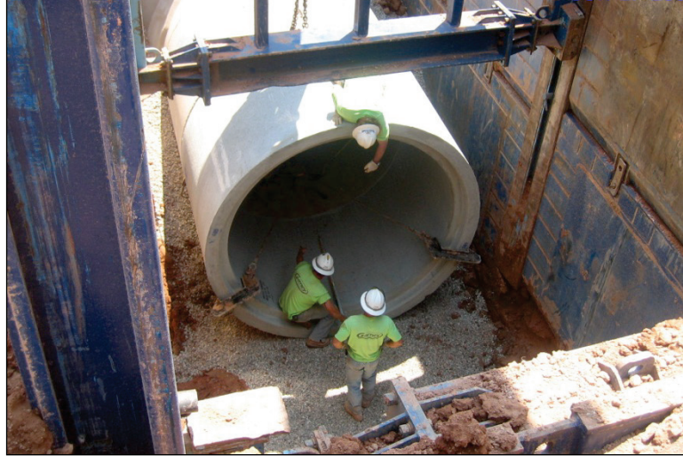
Figure 6.10. Open-trench excavation with shoring.
