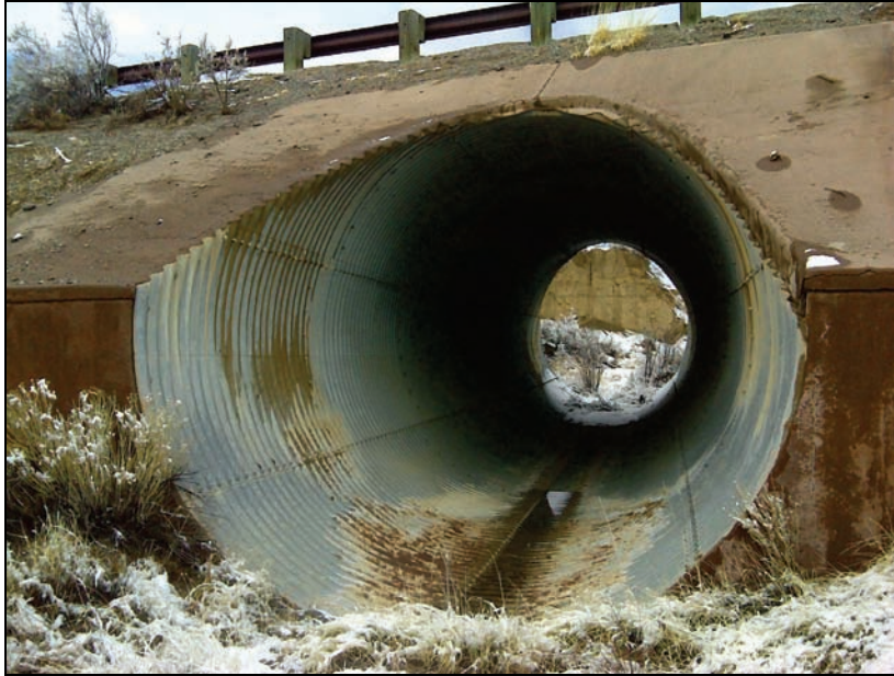
Figure 1.20. Structural plate culvert.
