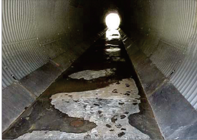
Figure 6.18. Invert repair of CMP using steel plating.
