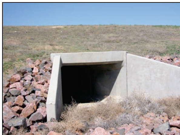
Figure 1.2. Typical concrete box culvert.
