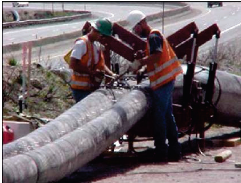
Figure 6.15. Deformed-reformed liner installation.
