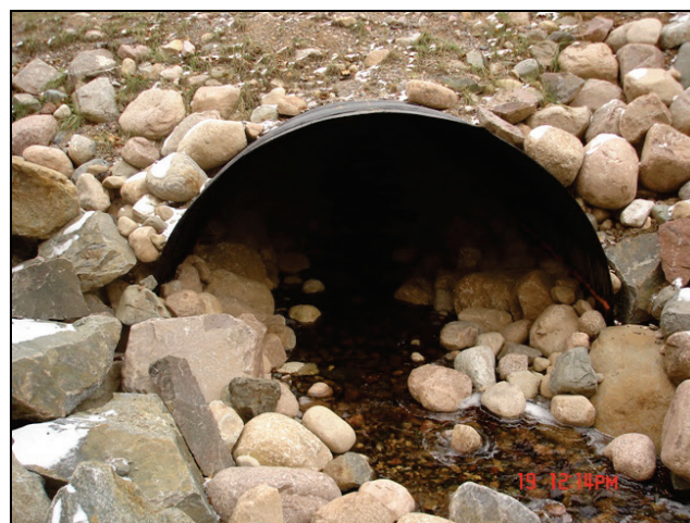
Figure 1.12. Embedded culvert (from WI DOT).
