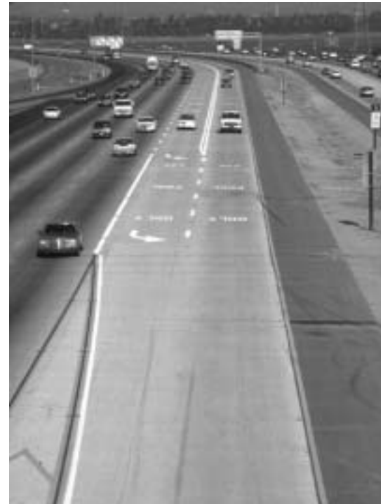
Figure 14. I-405 slip ramp and at-grade access, Orange County, California
