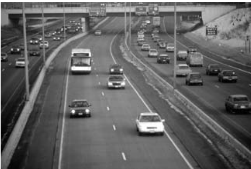
Figure 12. Concrete barrier on I-394 reversible lanes, Minneapolis
