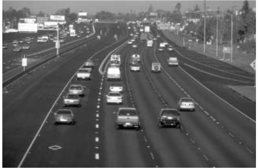
Figure 13. I-15 HOV lanes with slip ramp, Orange County, California
