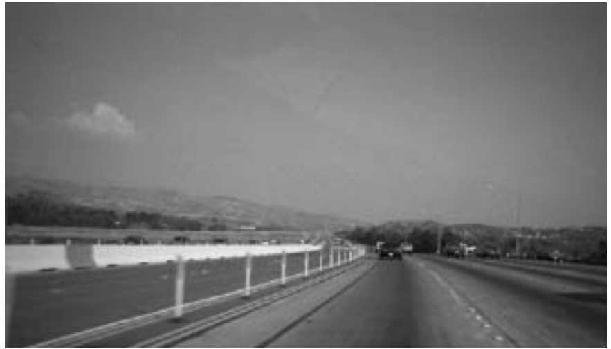
Figure 11. Tubular markers on SR 91
