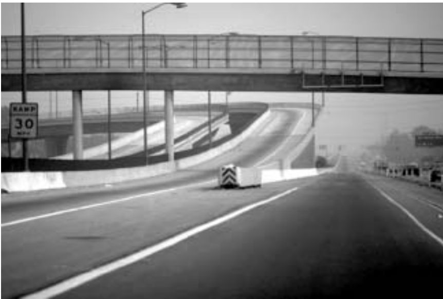
Figure 16. Grade separated HOV to highway flyover ramps
