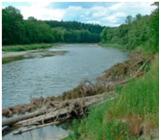
Figure 7.14 (left): River bed of the Thur River at Eggrank, Thurspitz, ZH, enhanced by structures, 2003 (photo: Floodplain Advisory Office SCZA).
