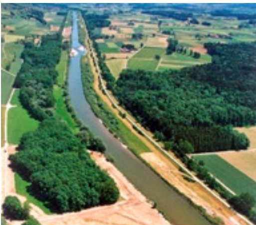
Figure 7.6: Small river widening in the Lichtenstein drainage canal adjacent to the Rhine River at Ruggell, 2005 (photo: A. Peter, Eawag).
