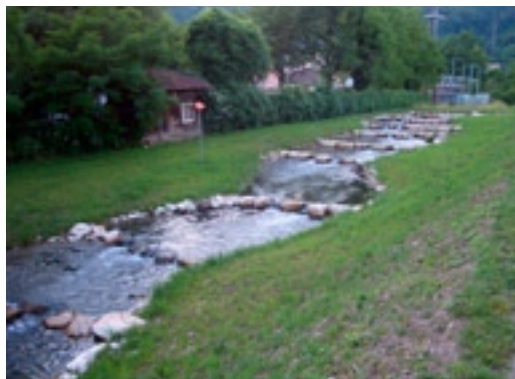
Figure 7.25: Bypass channel at the Aare River at Winznau, SO, 2005 (photo: A. Peter, Eawag, 2004).
