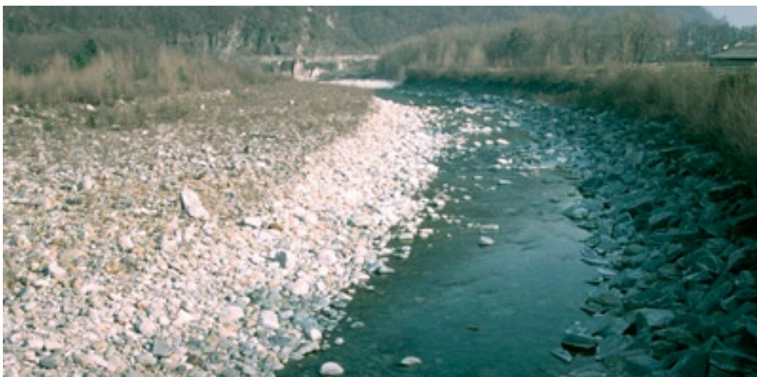
Figure 2.13: River bed erosion in the Melezza River, TI, 1997 (photo: L. Hunzinger, Schälchli, Abegg + Hunzinger).
