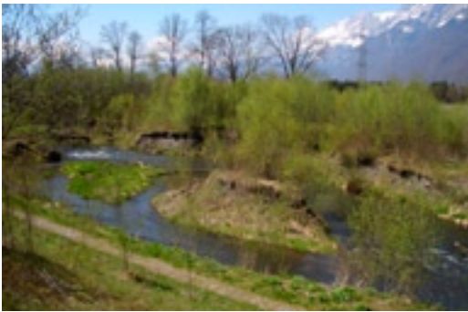
Figure 7.4: River widening at the Pascoletto River at Grono, GR, 2002 (photo: M. Hostmann, Eawag).
