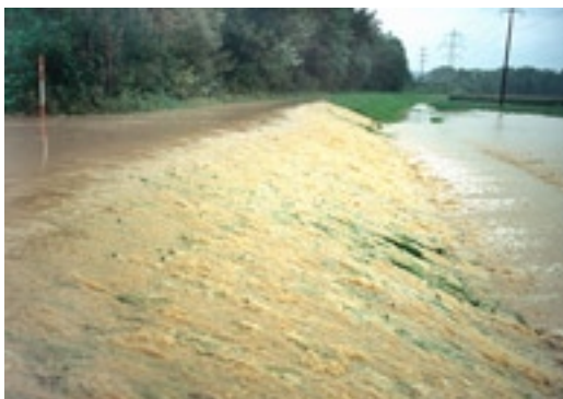
Figure 2.16: Flood effects at the Reuss River: spilt over dam at Joneh, AG, August 2005 (photo: B. Schelbert, Department of Construction, Traffic and Environment, Canton of Aargau, Division Landscape and Water).
