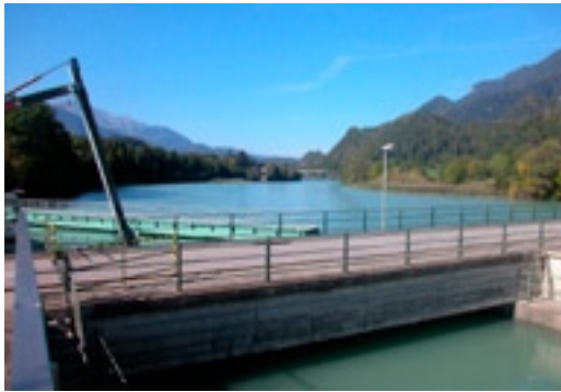
Figure 2.8: Dammed section in the Alpine Rhine River at Domat-Ems, GR, September 2003 (photo: A. Peter, Eawag).
