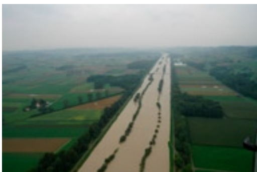
Figure 2.18: High flow at the Thur River at Uesslingen, TG. Due to sufficient flood protection no damages occurred here, August 2005 (photo: Police, Canton of Zurich).
