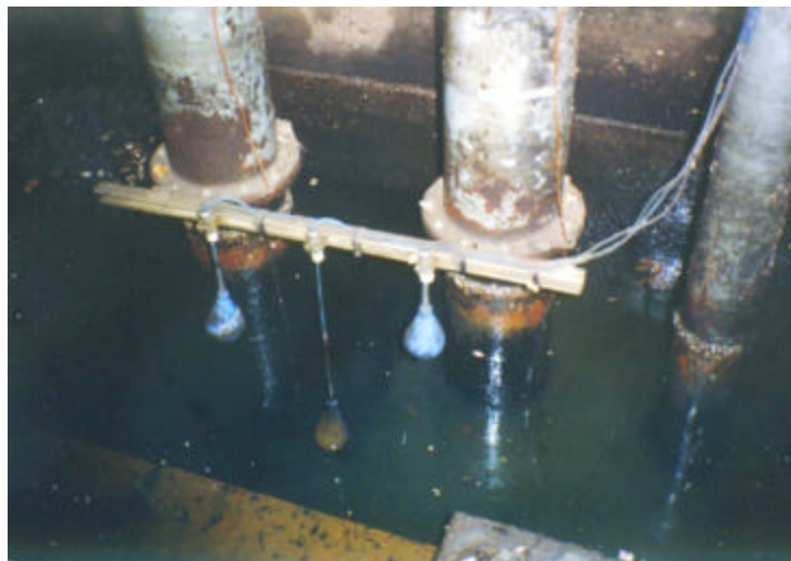
Figure 11-6. Tilting bulb switch
