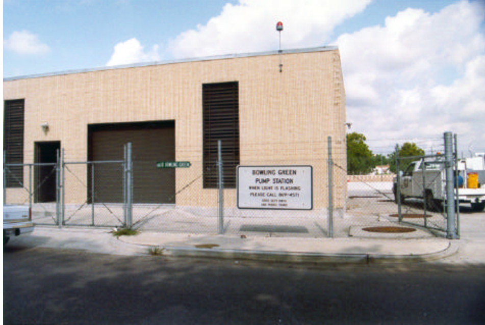
Figure 2-2. Highway stormwater pump house
