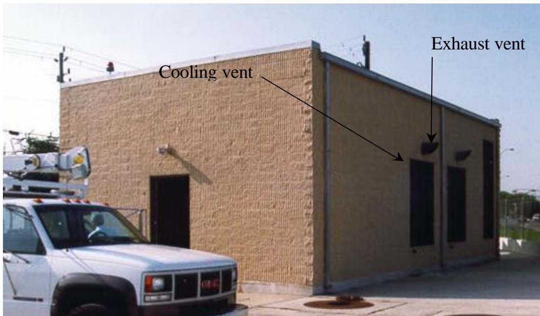
Figure 10-1. Typical pump house used by Texas DOT
