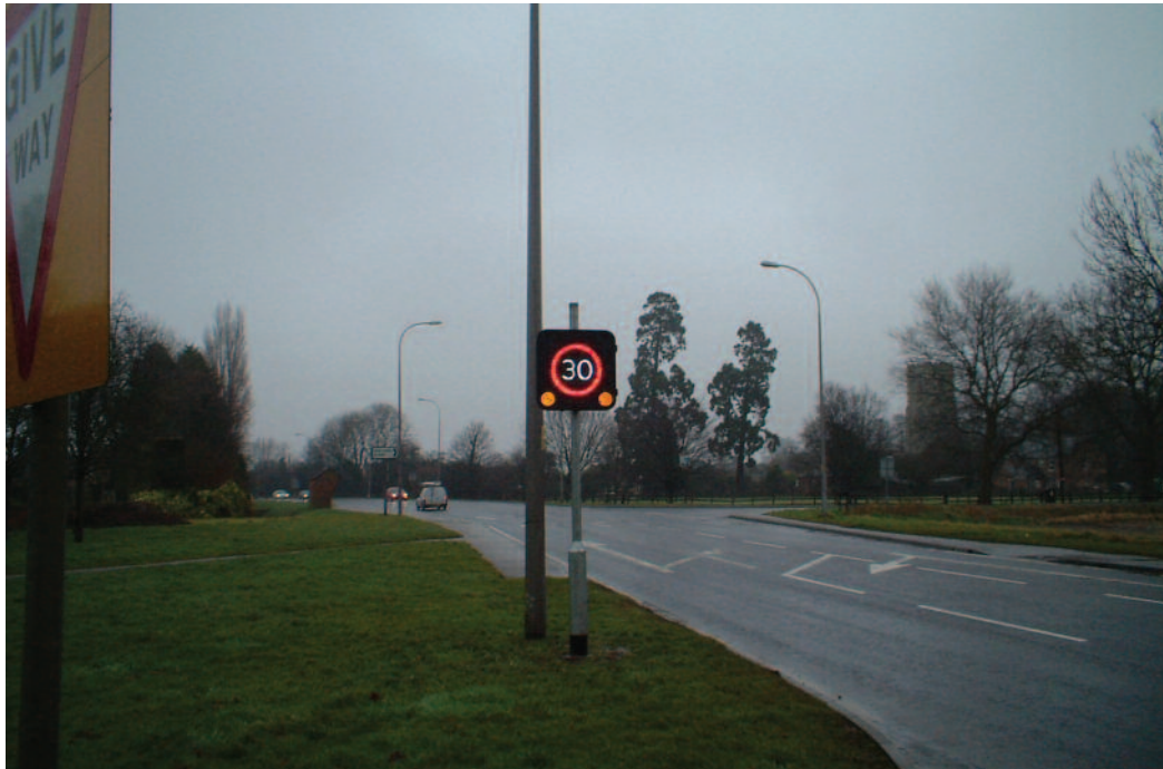
Figure 3.2 A 30 mph vehicle activated sign (VAS) at Sibsey in Lincolnshire, one of the rural demonstration projects (photo: Lincolnshire CC)
