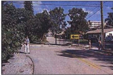
Ft. Lauderdale, FL - This diagonal diverter uses a narrow raised curb and landscaping to prevent through movements. Bicycle and pedestrian access is maintained along two cement-paved connections.
