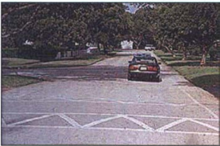
Ft. Lauderdale, FL - A 22-foot speed hump with zig-zag markings.
