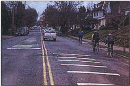
Portland, OR - This asphalt speed table uses leading horizontal stripe markings.
