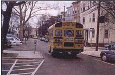
Cambridge, MA - These neckdowns slow vehicles approaching a bay of on-street parking.
