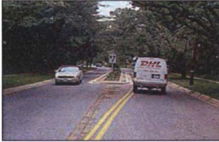
Montgomery County, MD - This center island narrowing is somewhat long. Visible on the pavement is the previous centerline before it was angled to guide motorists to the right of the island.
