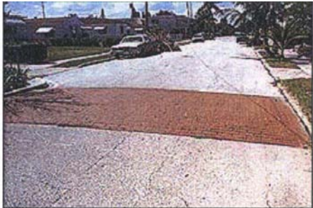
West Palm Beach, FL - This 12-foot hump is combined with Textured Pavement to enhance its visibility and speed-reducing effect.
