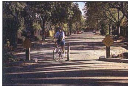
Palo Alto, CA - This closure uses two landscaped curb extensions and a single removable bollard to restrict motor vehicle access. The opening is wide enough to allow bicycle travel in both directions.
