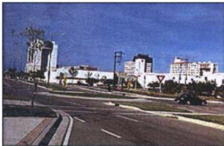
West Palm Beach, FL - This roundabout demonstrates the setback of the crosswalk from the circulating lane. This setback should allow at least one car to be able to pass the crosswalk and wait safely before entering the circulating lane once an adequate gap occurs.
