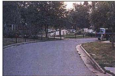
Boulder, CO - This diagonal diverter uses a wide raised, landscaped closure with a raised contour and a paved pedestrian/bicycle walkway connecting the two sides.
