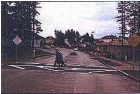
Beaverton, OR - This raised crosswalk uses asphalt and highly-visible paint.
