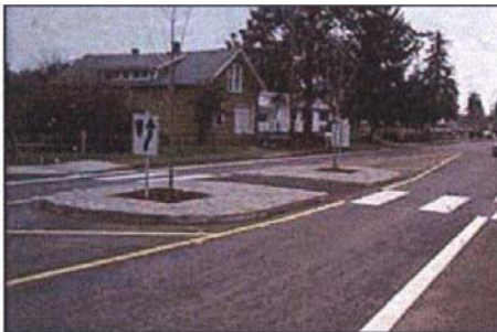
Portland, OR - This center island narrowing has hardscape but minimal live landscaping, minimizing maintenance costs.
