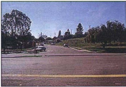
San Diego, CA - This median barrier uses a simple raised curb along the centerline of the major street. The pavement markings on the side street indicating that right-turns only are permitted are barely visible from this angle.
