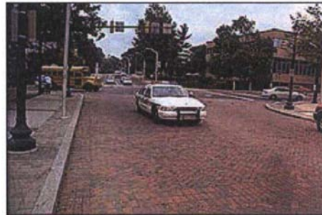
Seattle, WA - This textured pavement covers an entire downtown street block and the two endpoint intersections. It is also combined with neckdowns, though they are not pictured.
