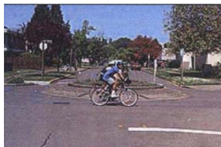
Seattle, WA - This traffic circle is located at a T-intersection, as indicated by the sign. A truck apron is included that allows trucks to make a left-turn, while passenger vehicles are discouraged from using the truck apron by the short lip at its edge.
