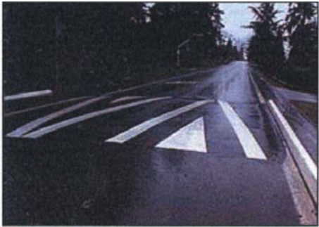
Bellevue, WA - This speed table is entirely asphalt with parabolic ramps.
