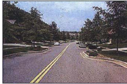
Montgomery County, MD - This choker uses slightly offset curb extensions to accommodate the residential driveways.
