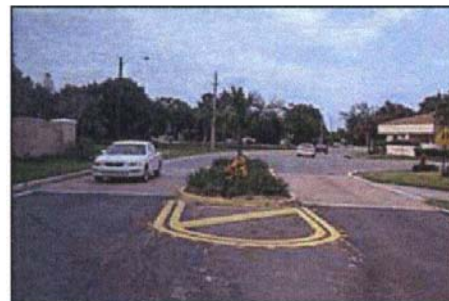
Ft. Lauderdale, FL - This center island narrowing is combined with Textured Pavement to provide a geway measure.
