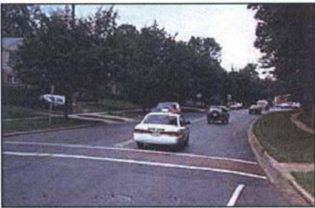
Montgomery County, MD - This raised crosswalk has tapers at the curbs to allow drainage to pass.
