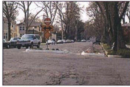
Sacramento, CA - Like the San Jose example, this half closure uses a short raised curb with a gap for bicycles. However, in this case the island is combined with a curb extension island that distinguishes the bicycle lane from the parking lane.
