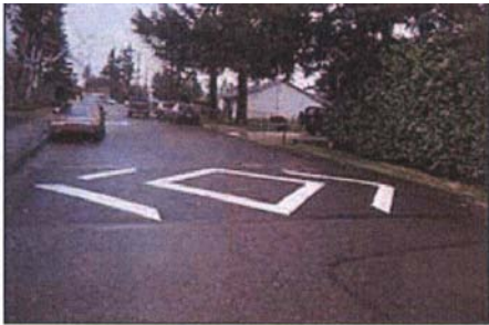
Portland, OR - This 14-foot speed hump uses a chevron marking pattern.
