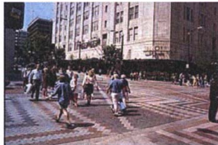
Seattle, WA - This textured pavement covers an entire downtown street block and the two endpoint intersections. It is also combined with neckdowns, though they are not pictured.
