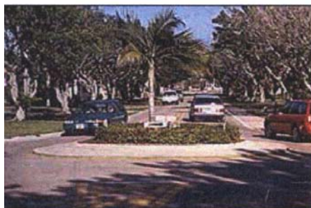
Ft. Lauderdale, FL - This traffic circle has a larger truck apron. Splitter islands and yield lines have been striped at each approach.
