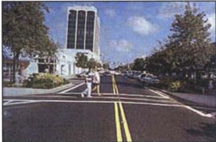
Cambridge, MA - These neckdowns slow vehicles approaching a bay of on-street parking.
