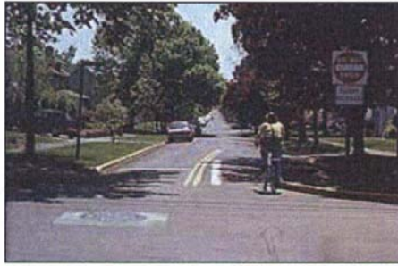
Eugene, OR - This half closure does not include a gap on the right side for bicycles, but rather is truncated to allow bicycles to pass on the left. This also allows enough width for fire and police vehicles to easily enter when responding to an emergency.
