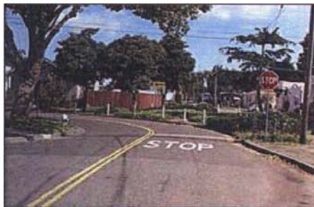
Berkeley, CA - This diagonal diverter uses ground cover landscaping in lieu of trees.
