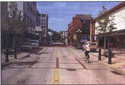
Eugene, OR - This raised crosswalk uses a unique pattern of concrete and brick Bollards are provided to assist visually-impaired pedestrians detect the beginning of the crosswalk.
