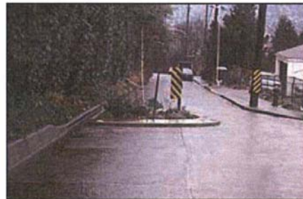
Seattle, WA - This urban residential intersection uses an island to deflect the through street.
