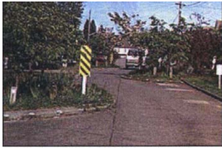
Seattle, WA - These chicane islands extend out to the roadway centerline, creating a highly deviating path.
