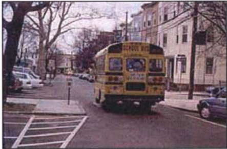
Cambridge, MA - These neckdowns slow vehicles approaching a bay of on-street parking.
