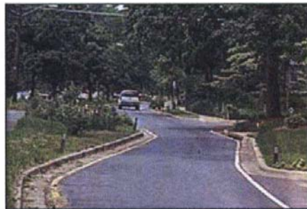
Montgomery County, MD - Here is a one-way chicane, created by a deviating curb-and-gutter.
