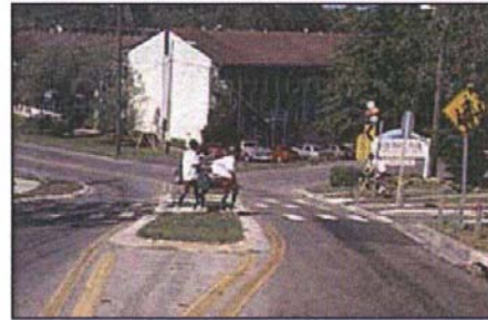
Portland, OR - This center island narrowing is combined with two crosswalks.
