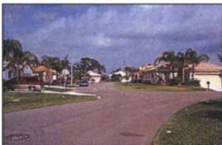
Deerfield Beach, FL - Again, these roadways have no curbs, so modification is relatively inexpensive.
