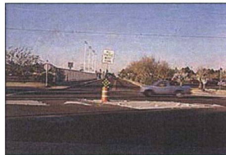
Phoenix, AZ - This median barrier allows both right - and left-turns out of the side street but prohibits through movements by explicitly channeling the left-turn movement.
