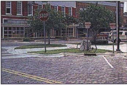
Gainesville, FL - This textured pavement is combined with diagonal parking and neckdowns at the corners.
