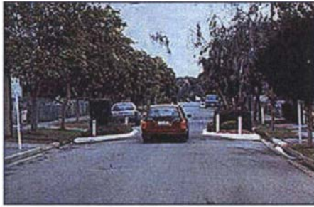
Howard County, MD - This is a one-lane choker. Vehicles on one side yield to vehicles from the other side until the queue is cleared, just as on one-lane bridges.
