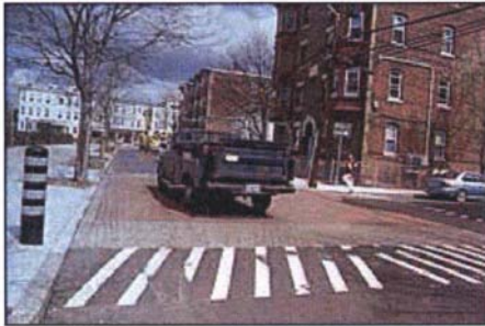
Montgomery County, MD - This raised crosswalk has tapers at the curbs to allow drainage to pass.
