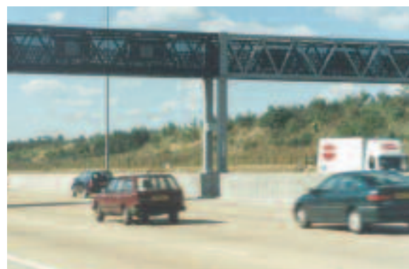
Concrete motorway divider.
