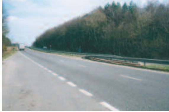
After safety fencing installed.
