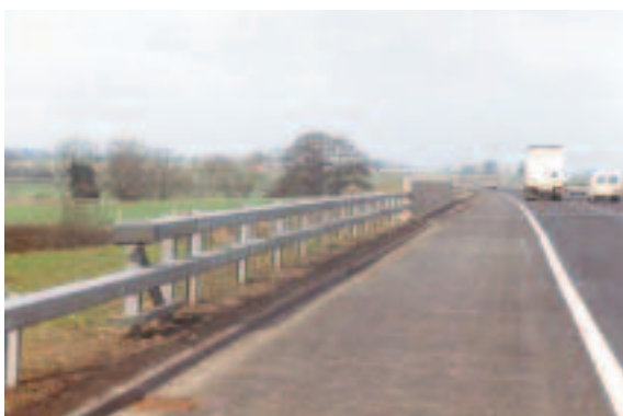
Hollow box section and concrete barrier bridge parapet.
