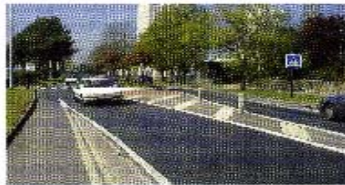
This busy boulevard in Nantes, which was once a dual two-lane road, has been redesigned to limit speeds and provide more space and increased safety to non-motorised users.
