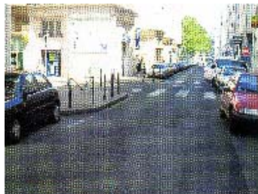
Simple measures such as pavement extensions can be standardised and scheduled in the PDU.
