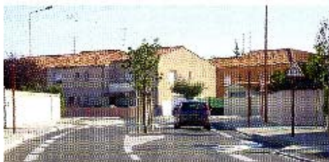
Speeds can be influenced in many ways, like this chicane on a neighbourhood road.
