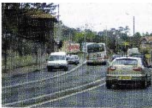
Another example of the redesign of a major road, which reduces the road from a dual two-lane carriageway to a single lane in each direction, whilst providing an exclusive way in the centre for public transport and a kerb-side cycle lane (Lyon metropolitan area).
