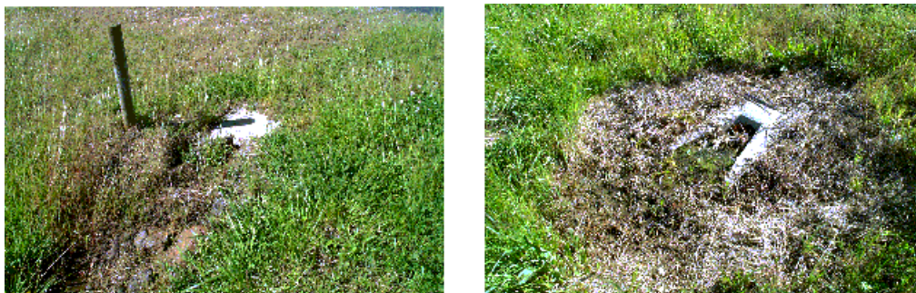
Figure 5.5: Subsurface drain outlets
