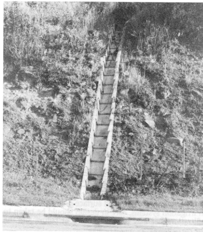
Figure 6.7: Open chute (after NAASRA, 1986)
