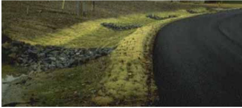
Figure 8.1: Rock check dams
