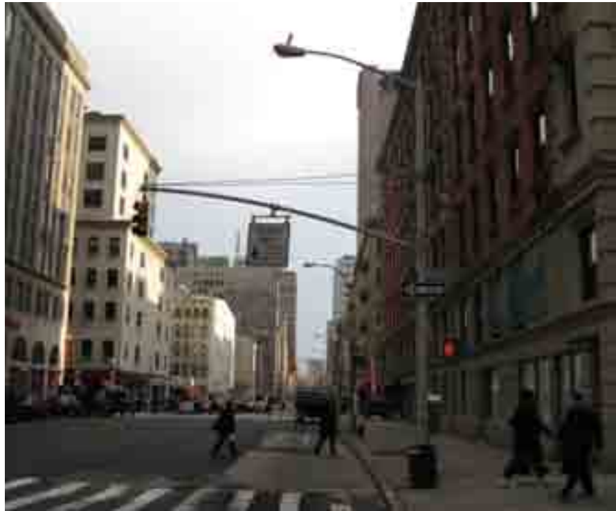
Type M-2 Traffic Signal Pole with standard luminaire: Murray Street, Manhattan
