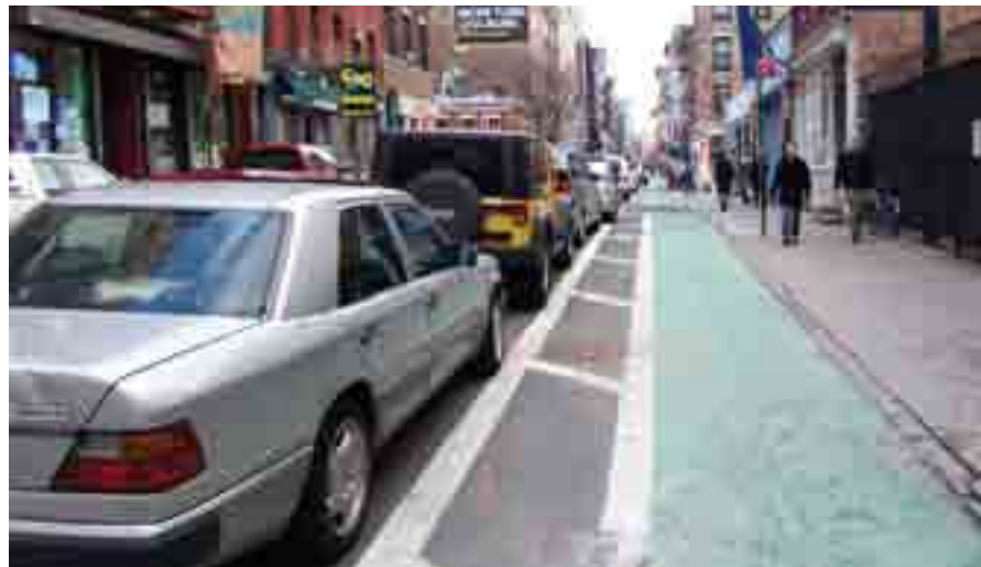
One-way, parking-separated bike path on a crosstown street: Grand Street, Manhattan
