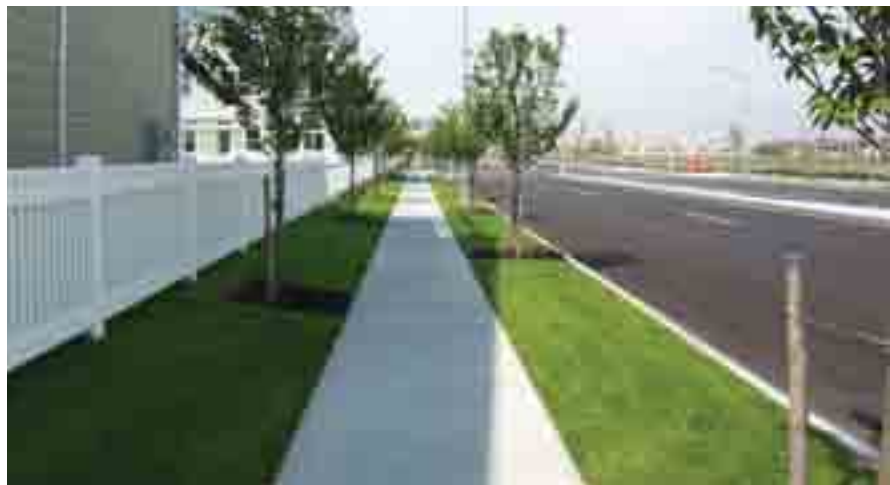
Concrete ribbon sidewalk: Rockaway Beach Boulevard, Queens
