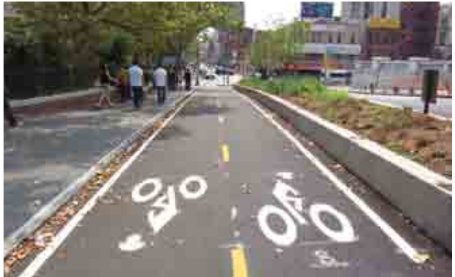
Two-way bike path separated with landscaped median: Canal Street, Manhattan
