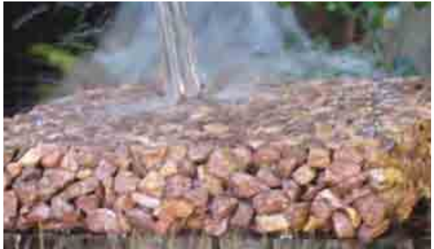
Voids in between stones allow water to pass through (note: for demonstration purposes, this example shows a clear resin, not asphalt, to bind the aggregate particles)
