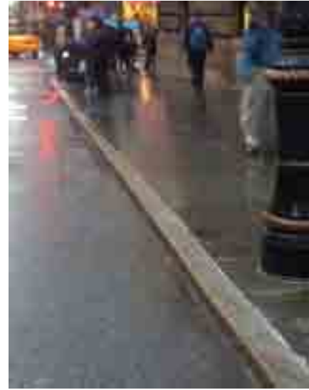
Saw-finish granite curb shown with historic bluestone sidewalk: Madison Avenue at East 51st Street, Manhattan
