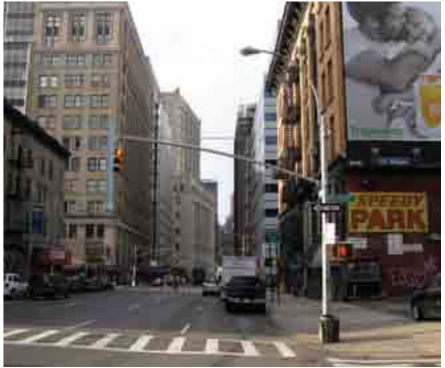
Type M-2 Traffic Signal Pole with standard luminaire: Lafayette Street, Manhattan
