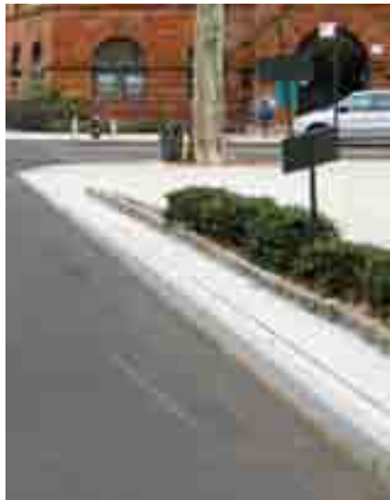
Typical untinted concrete curb with steel facing: West 114th Street and Morningside Avenue, Manhattan
