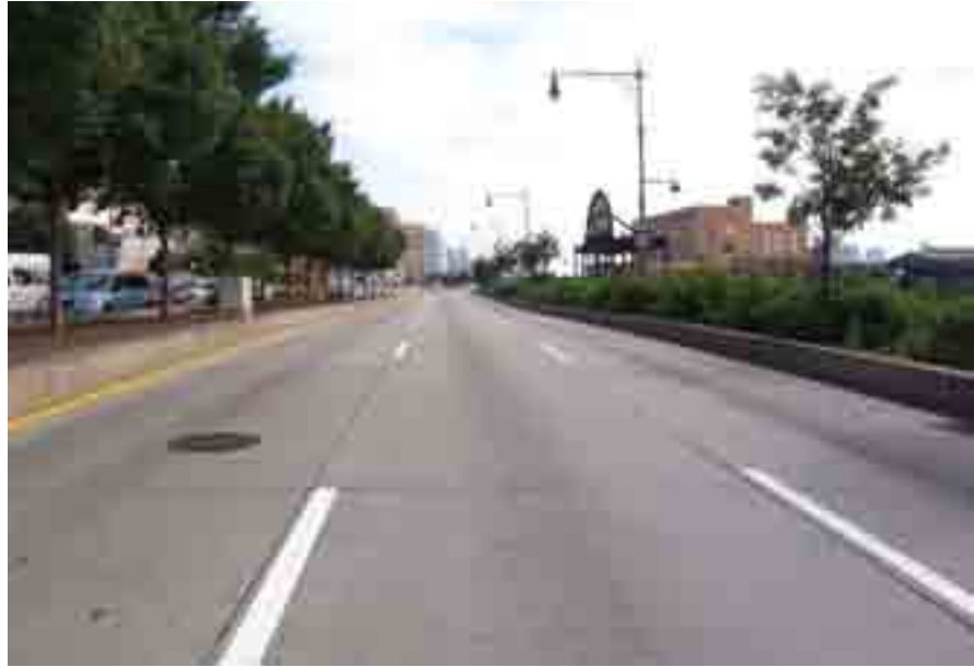
Typical concrete roadbed: West Side Highway, Manhattan
