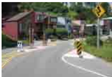
Chicane at entry to residential neighborhood: San Francisco, California (Credit: SF MTA)
