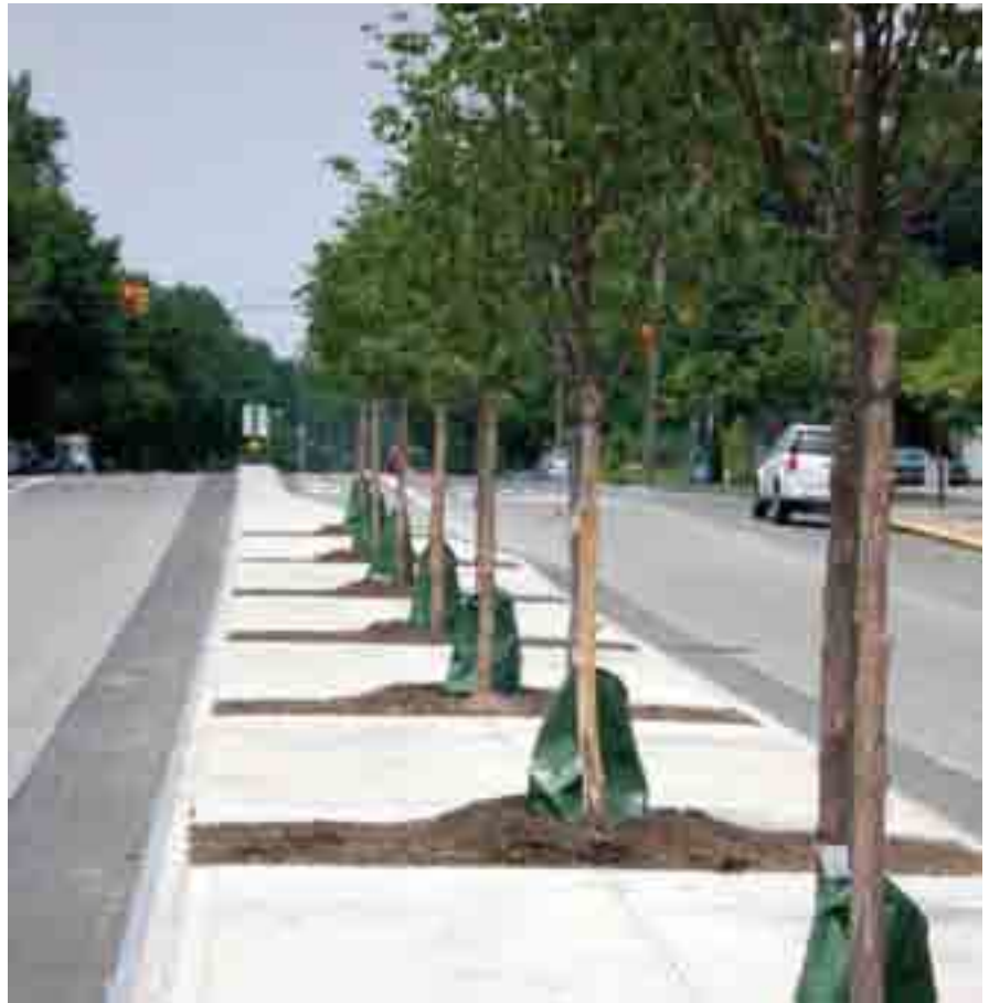
Individual tree pits in a median (deep irrigation bags are secured to tree bases); Page Avenue, Staten Island (Credit: NYC DPR)
