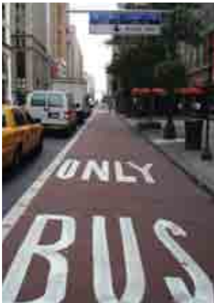
Red, curb-aligned, on-street busway with "soft separation" from traffic: 34th Street, Manhattan
