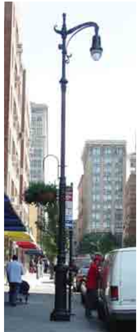
Historic Teardrop luminaire and Type F pole: East 8th Street, Manhattan
