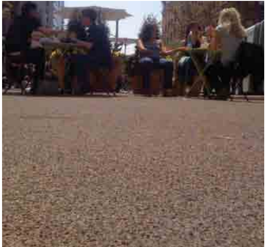
Resin-bound gravel treatment applied to existing asphalt roadway to create a temporary pedestrian plaza: 9th Avenue at West 14th Street, Manhattan
