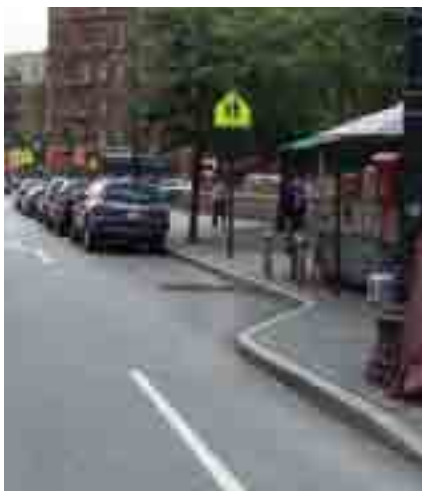
Curb Extension: Seventh Avenue, Manhattan
