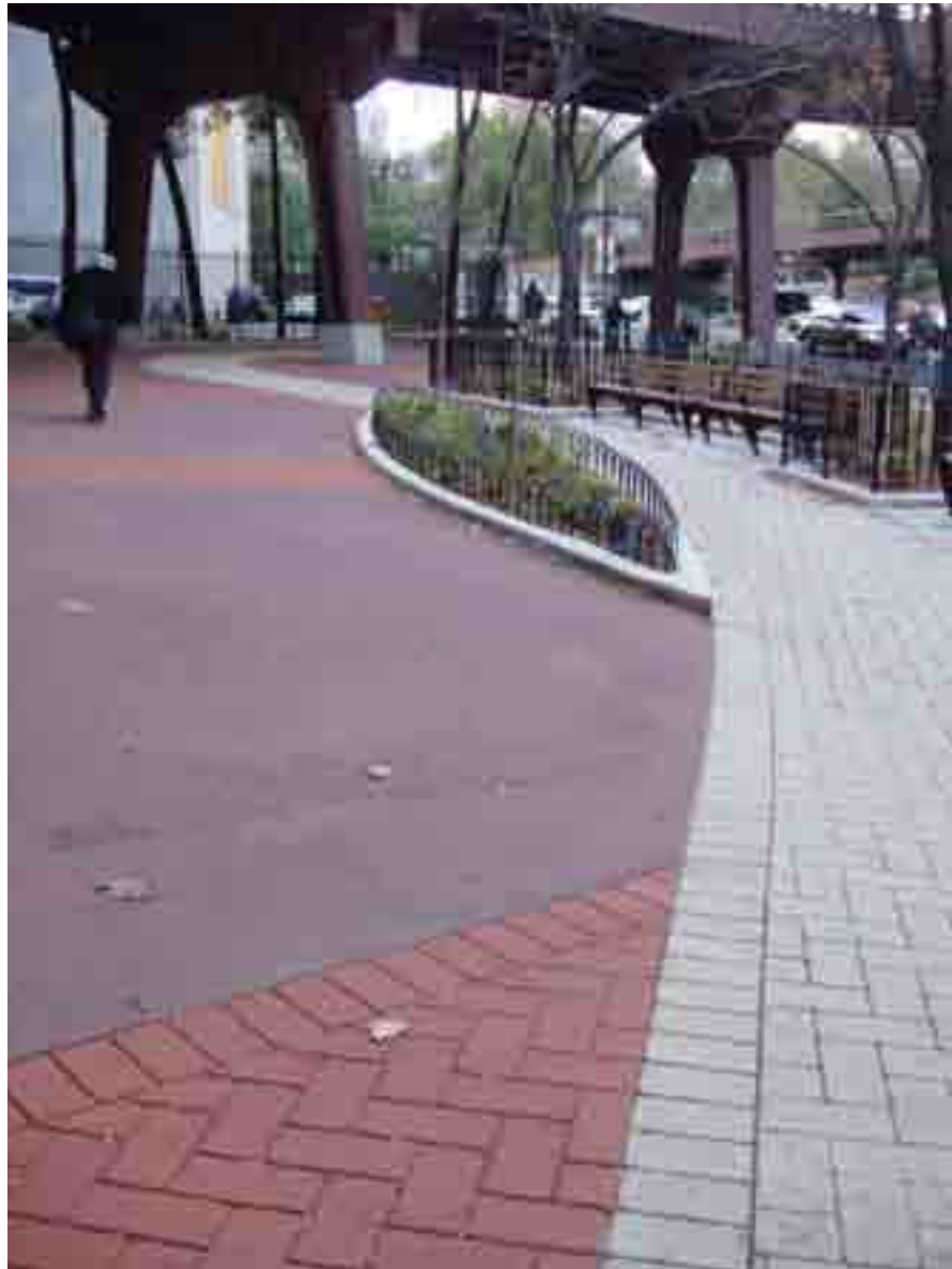
Imprinted asphalt in a plaza: Drumgoole Plaza (Gold Street at Frankfort Street), Manhattan
