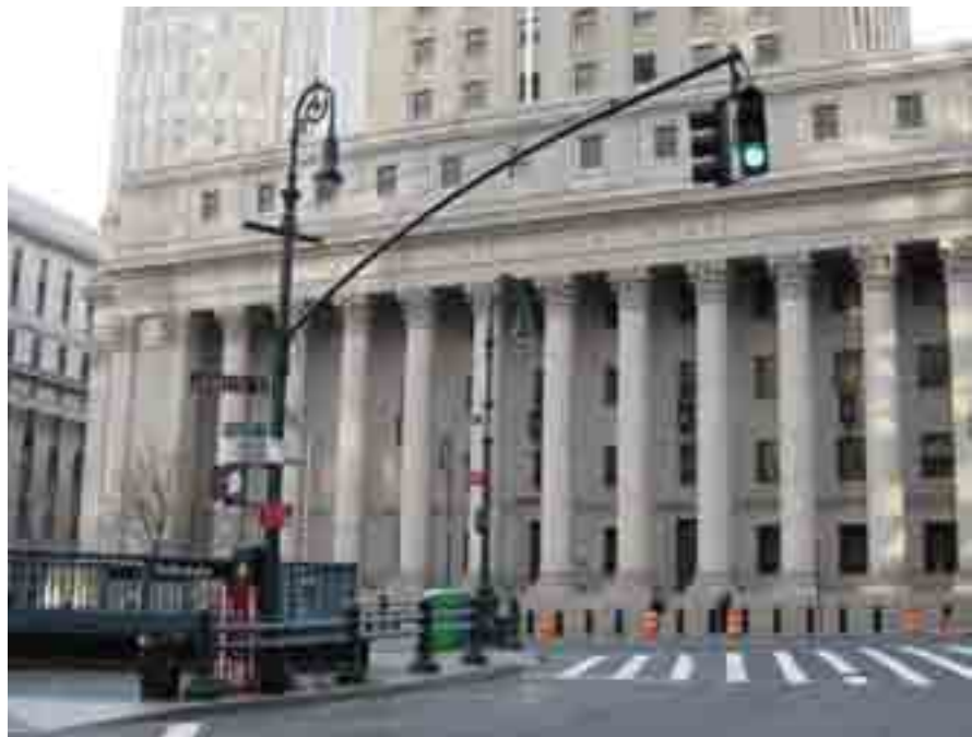
Type M-2 Traffic Signal Pole with historic luminaire: Warren Street, Manhattan
