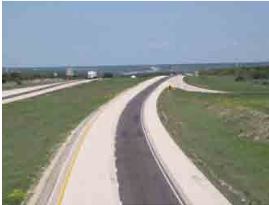
Highway showing left side paved with high-albedo asphalt and the right side paved with conventional asphalt: Interstate 10, West Texas (Credit: The Citizen Scientist, April 16, 2004)
