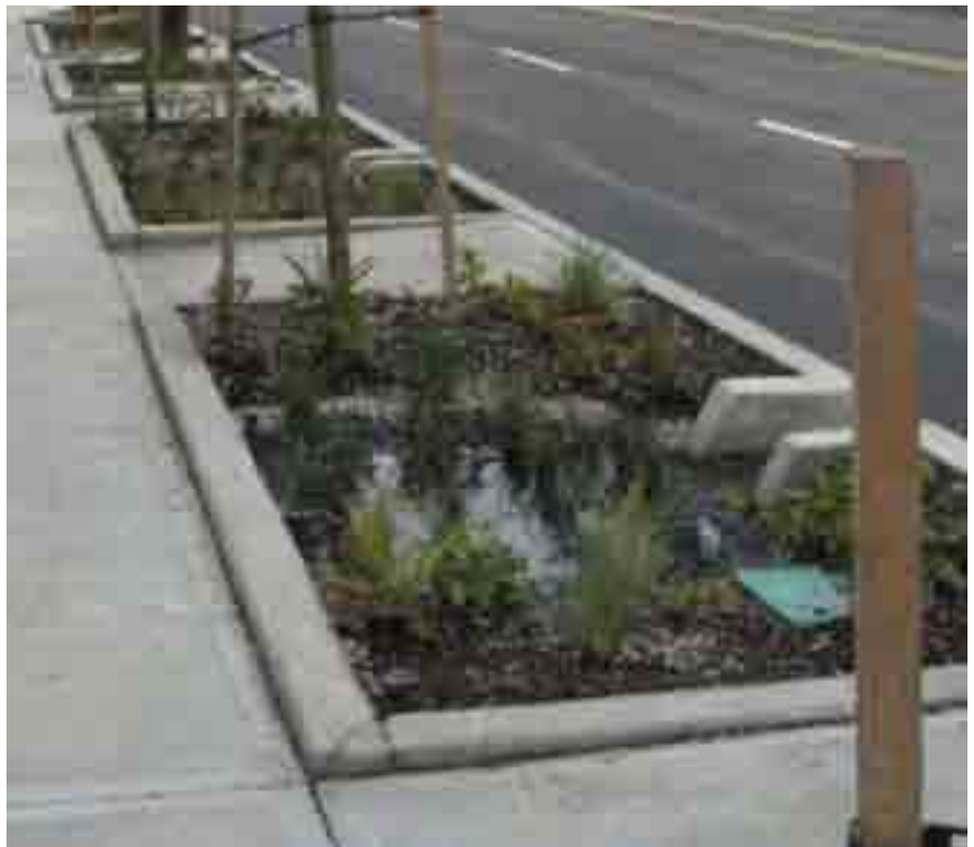
Stormwater–capturing tree pit with plantings: San Francisco (Credit: San Francisco Planning Department)
