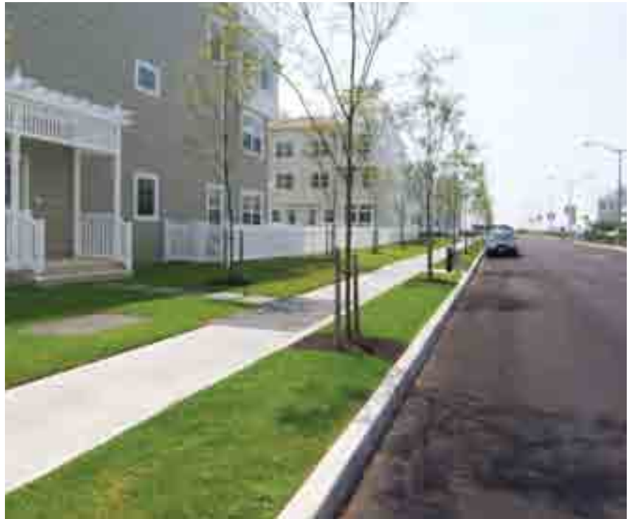
Typical concrete curb: Beach 73rd Street, Queens
