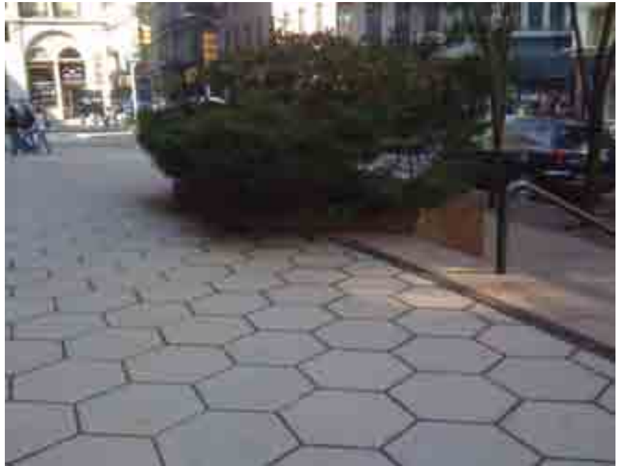
Hexagonal concrete pavers in a privately owned plaza: White Street at Broadway, Manhattan
