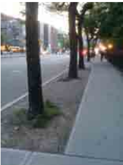
Connected tree pits with uncovered trench: West Houston Street, Manhattan
