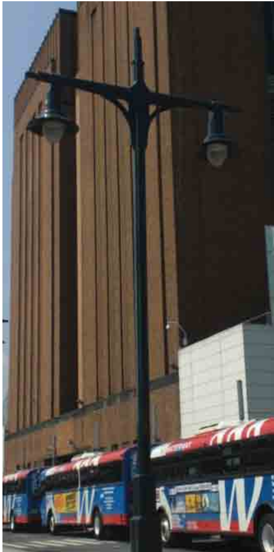
Historic Shielded Teardrop luminaire and TBTA Pole: 40th Street, Manhattan
