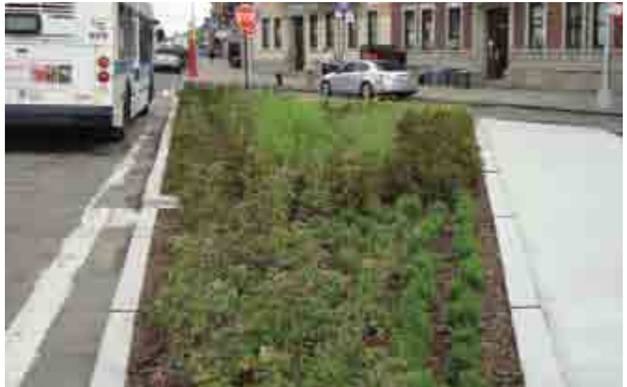
Street swale: Church Street at 35th Street and 14th Avenue, Brooklyn
