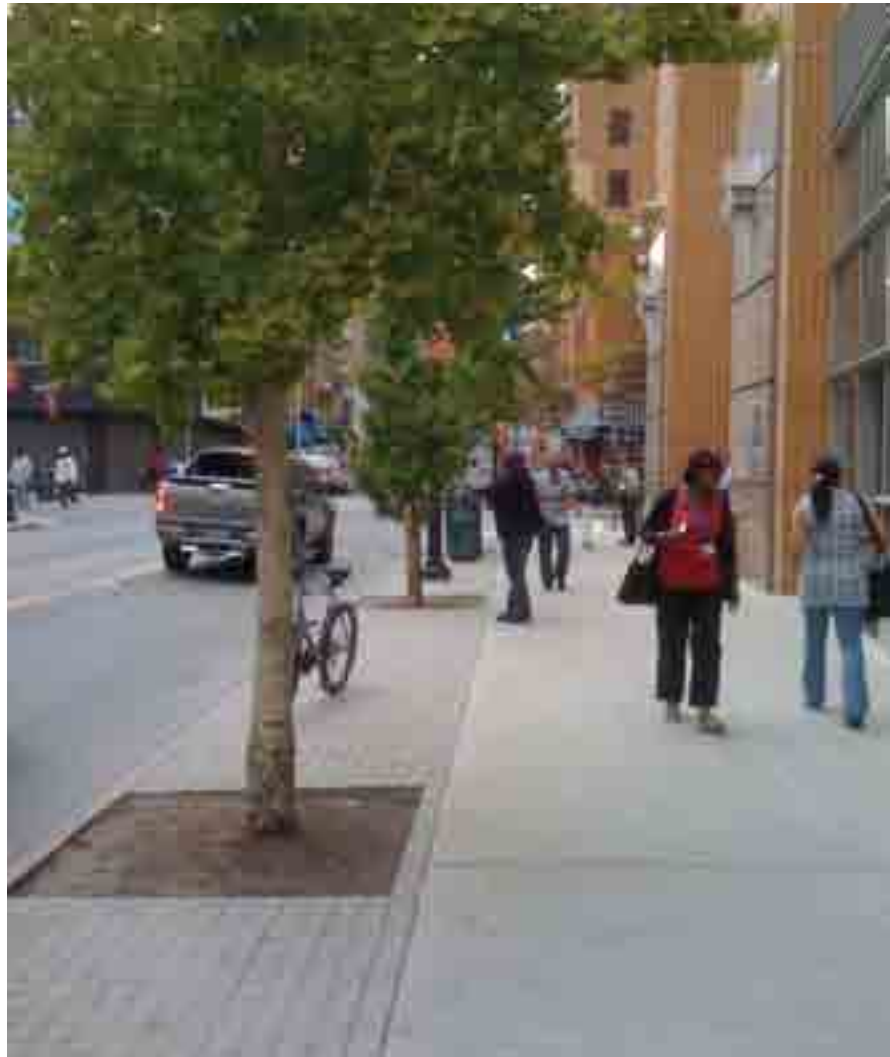
Square asphalt pavers in a furnishing zone: Willoughby Street at Duffield Street, Brooklyn
