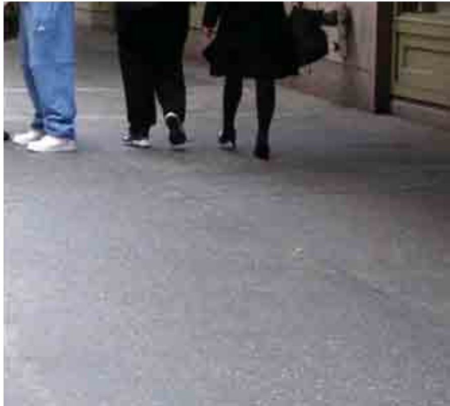
Tinted concrete sidewalk with light-colored exposed aggregate (note: this example does not include the required "simulated saw-cut joint" scoring pattern): 42nd Street at Grand Central Terminal, Manhattan
