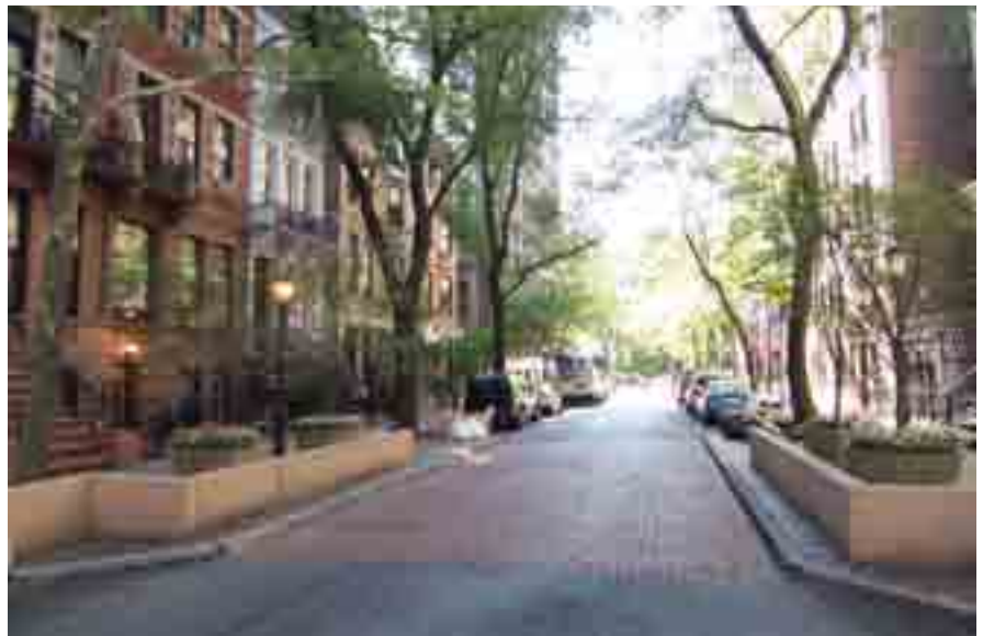
Mid-block narrowing (Note: use of walls is not recommended by this manual); West 94th Street, Manhattan
