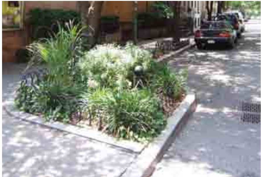
Curb extension with planted area: Mulry Square, Manhattan
