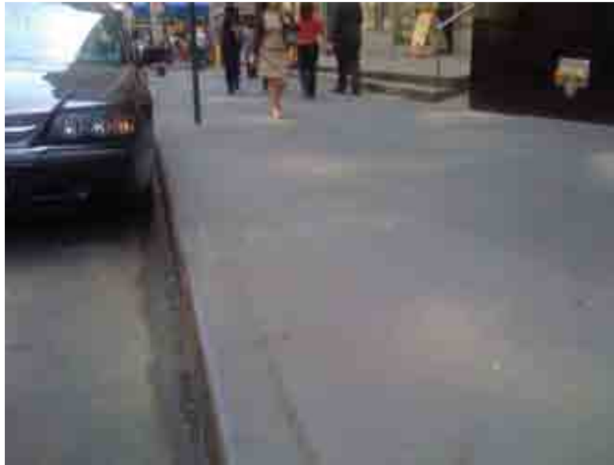
Typical tinted concrete curb with steel facing: Beaver Street at Hanover Street, Manhattan
