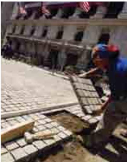
Modular cobblestone installation: Broad Street at Wall Street, Manhattan (Credit: Eurocobble®)
