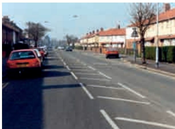
Fig. 10.2 Hatched road markings
