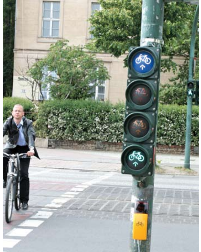
Figure 27. Bicycle traffic signals control bicycle traffic movements at signalized intersections in Potsdam, Germany. (Note: A blue plaque placed in the highest signal lens is not intended to control bicycle movements.)
