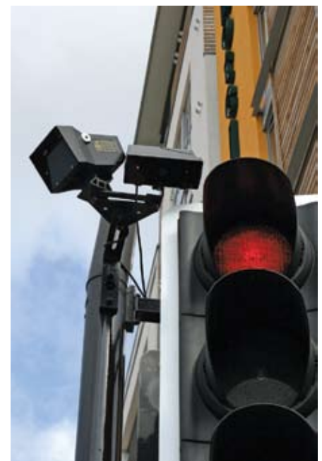
Figure 11. Automated pedestrian sensors for adapting signal timing for pedestrians in Bristol, United Kingdom.
