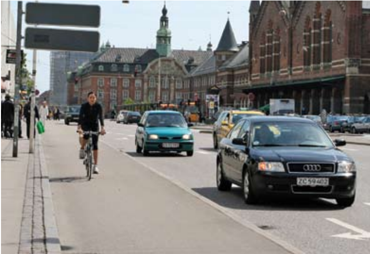
Figure 20. Cycle track in Copenhagen, Denmark.
