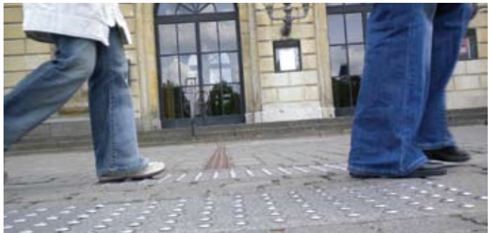
Figure 18. Tactile sidewalk strips leading to front door of public building in Copenhagen, Denmark.
