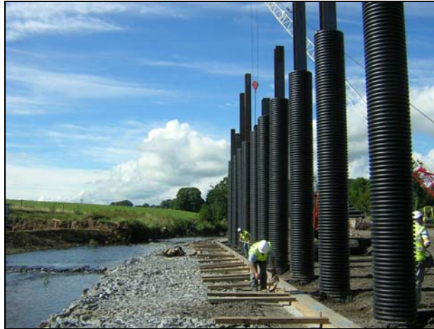
Figure 9.2 Use of plastic pipe sleeves around H-piles
