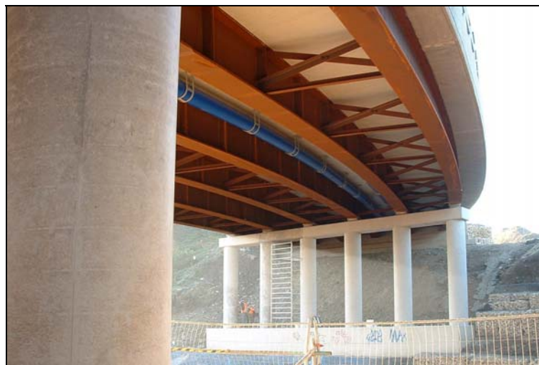
Highfield Lane Bridge (Photo by courtesy of Rotherham Metropolitan Borough Council)
