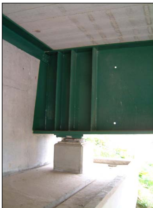
Overbridge on BNRR (Photo by SCI)
