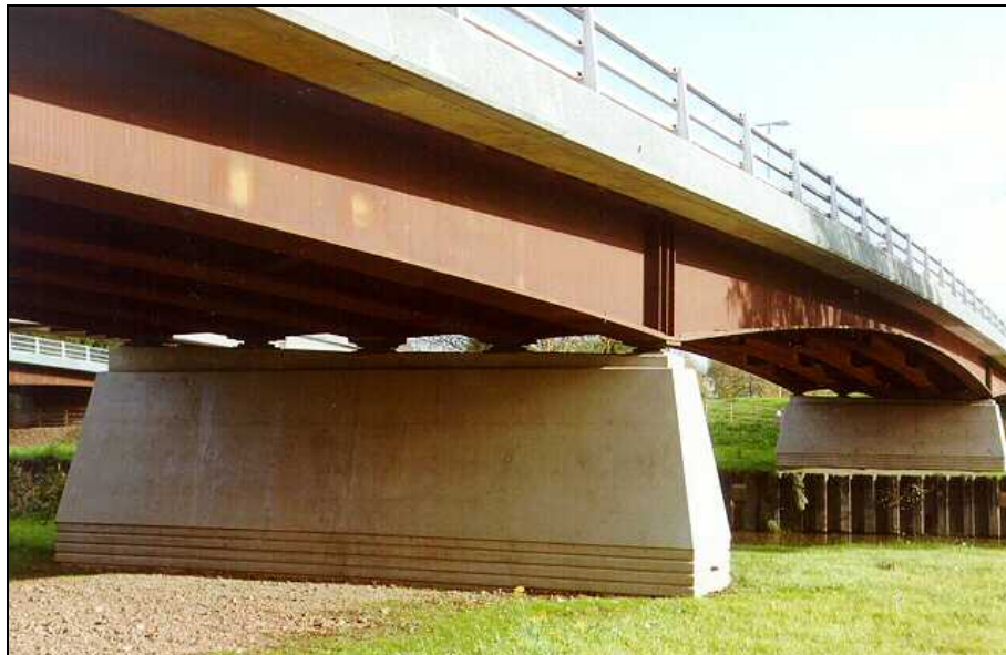
Westgate bridge, Gloucester (Photo by courtesy of Corus)
