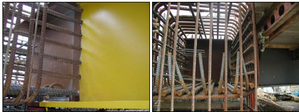
Figure 9.8 Reinforcement in endscreen wall
