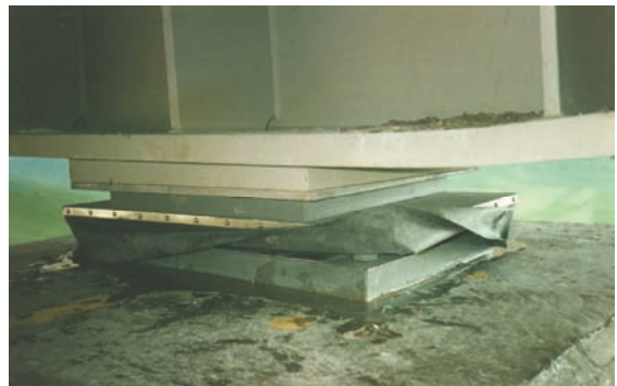
Figure 3 Guided bearing (with skirt)
