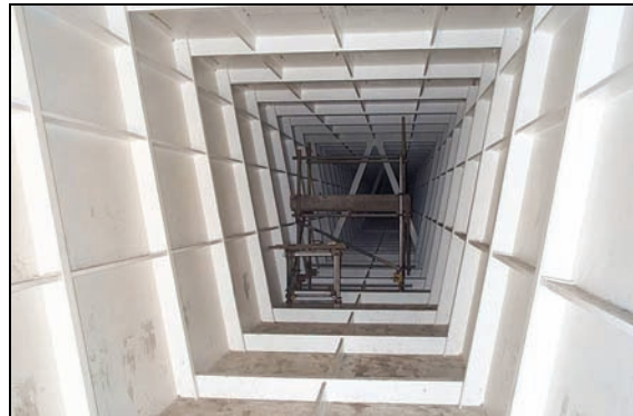
Figure 1 Internal view of a steel box girder showing use of longitudinal stiffeners
