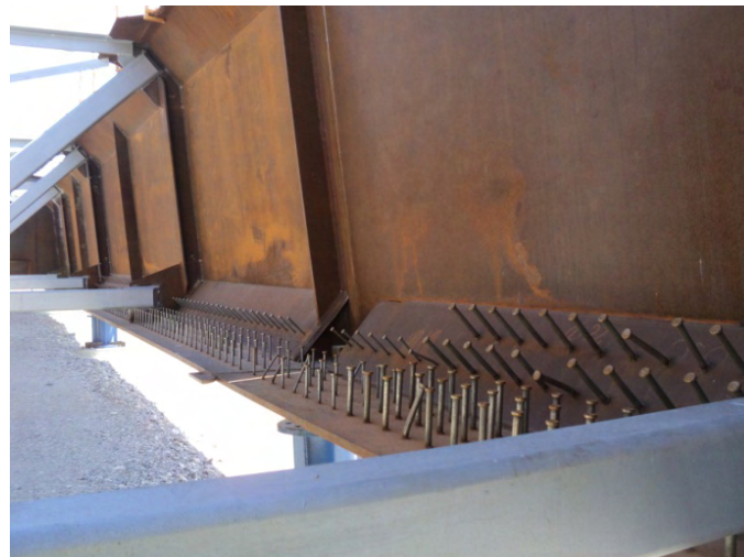
Fig. 6.26 View of the lower flange connection of a steel girder
