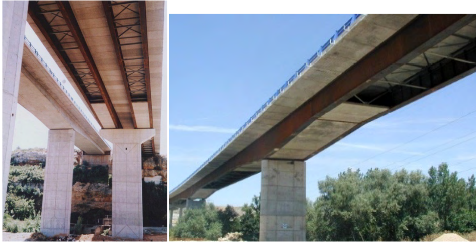
Fig. 6.10 Two examples of road composite bridges with double composite action in hogging areas
