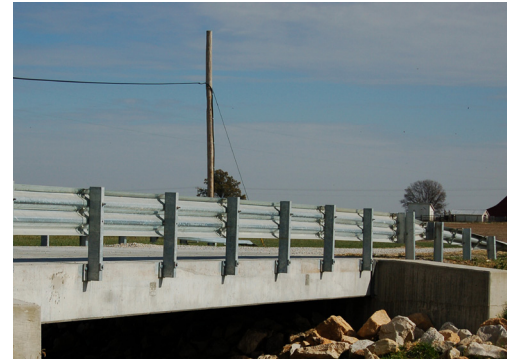
Audrain County Bridge 336
