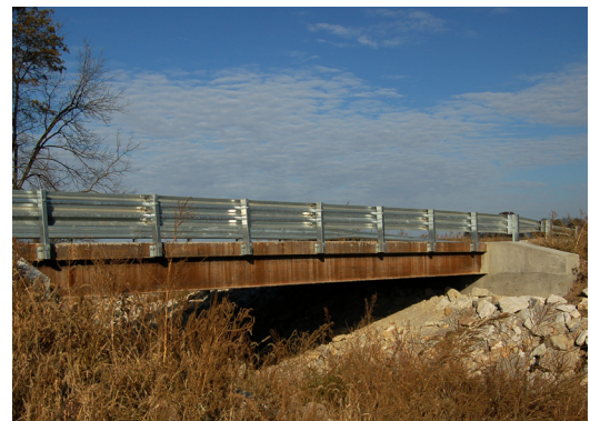
Audrain County Bridge 411
