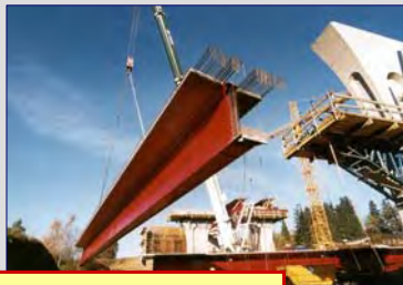
installation by crane
