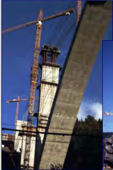
cantilever erection of the arch
