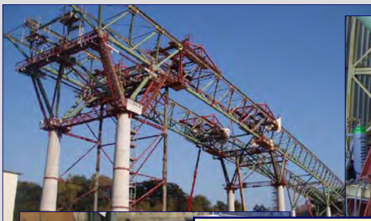
steel trusses with hollow sections and cast iron nodes
