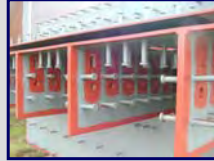
joint with overlapping steel plates and headed studs
