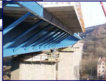
concrete deck with partially prefabricated concrete elements
