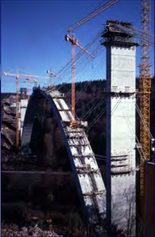
cantilever erection of the arch
