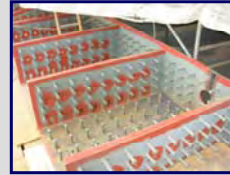
joint with overlapping steel plates and headed studs
