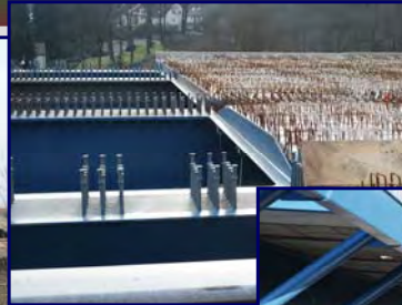
concrete deck with partially prefabricated concrete elements
