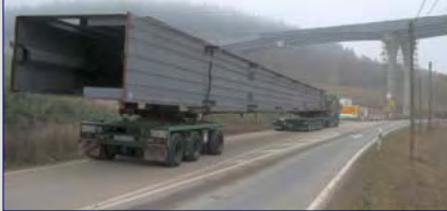
transportation of steel girders on site
