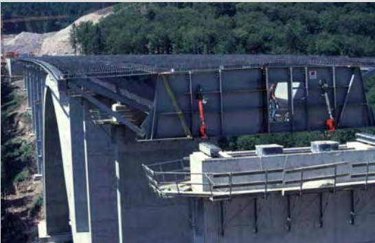
Bridge girder during launching
