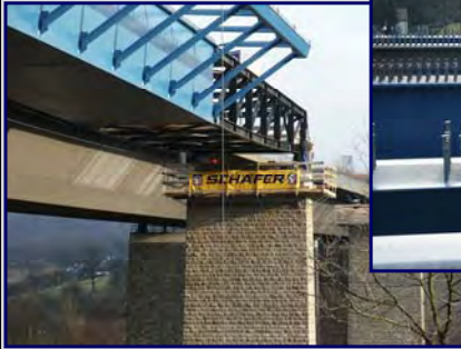
launching of the bridge with partially prefabricated concrete elements
