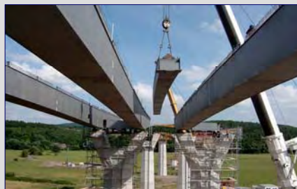
erection of steel girders by cranes
