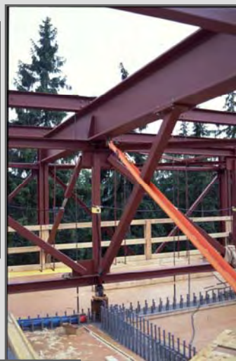
Bridge Wilde Gera
