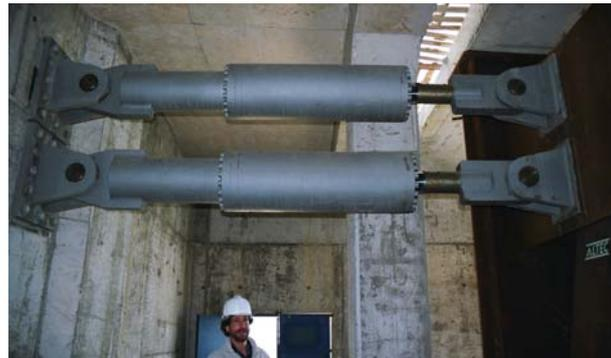
**Fig. 4:** Underneath view during launching    **Fig. 5:** Longitudinal viscous damper-shock transmission
