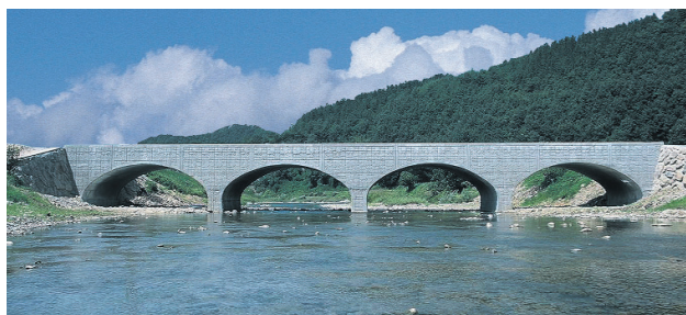
Illustration 4: Multiple Span Box Culvert
