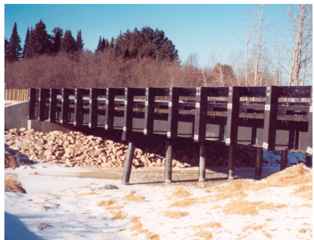
Illustration 2: Steel Superstructure with Treated Timber Deck and Rails
