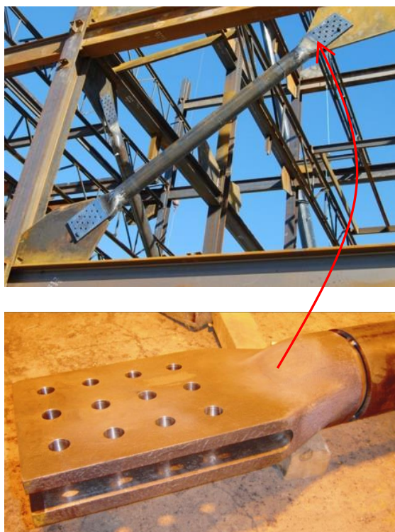
Figura 4-31. Conexión Cast ConneX High-Strength Connector ( http://www.castconnex.com )
