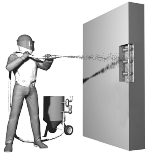
Fig. 4—Final surface cleaning.
