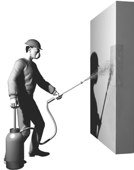
Fig. 9—Spray application of curing compound.
