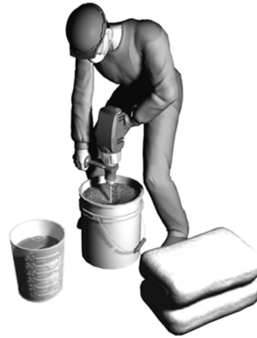
Fig. 7—Typical equipment to mix materials.
