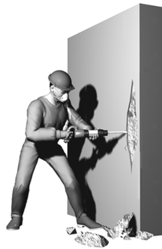
Fig. 2—Bulk concrete removal.
