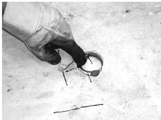
Fig. 13—Type 2A anode placed in hole with patching material.
