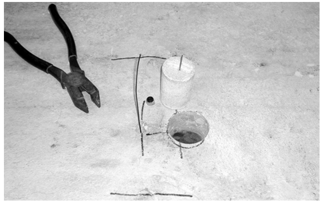
Fig. 11—Secondary hole with reinforcing steel connection.
