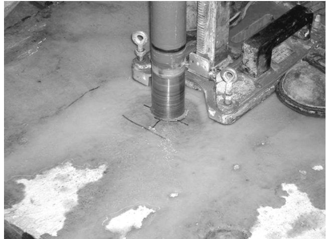
Fig. 10—Coring hole for anode.
