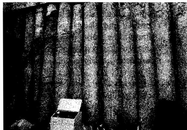
Figure 21. Completed tangent pile wall.
