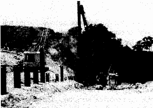
Figure 18. Driving soldier piles.
