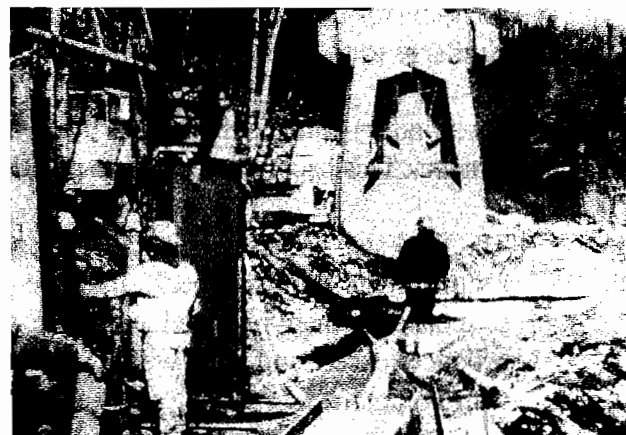
Figure 25. Hydraulic clam shell for excavation.
