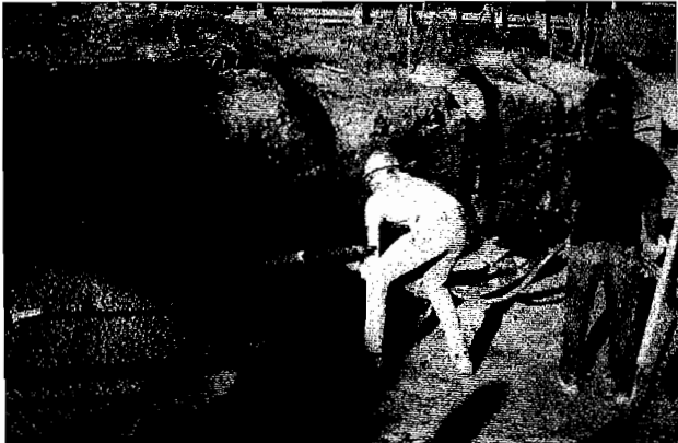
Figure 41. Grouting of soil nail.
