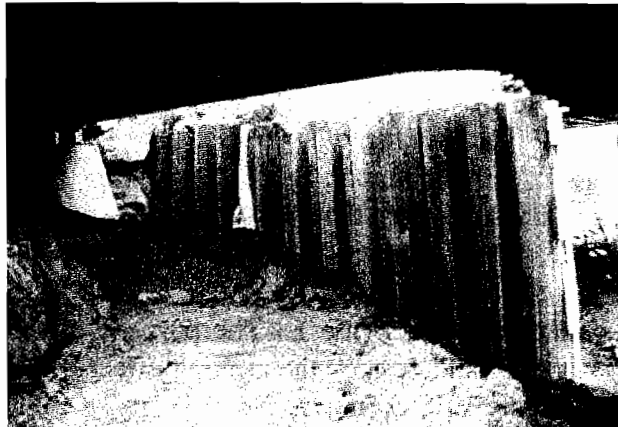
Temporary sheet-pile wall
