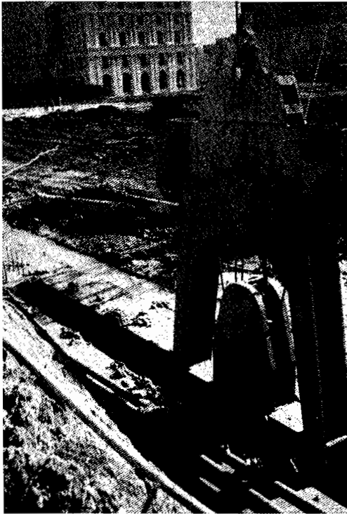
Figure 22. Conventional grab bucket for slurry (diaphragm) wall construction.
