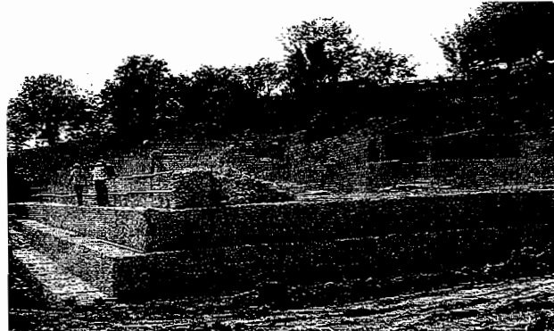
Construction of gabion wall
