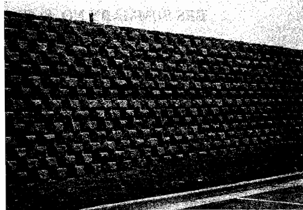
Completed modular block wall
