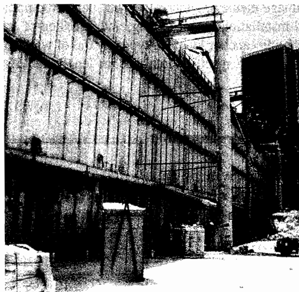
Completed soil mixed wall
