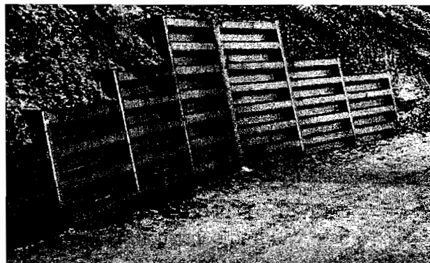
Completed metal bin wall
