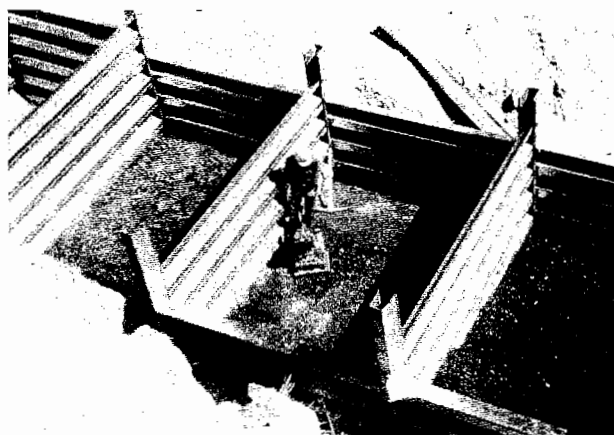
Figure 9. Compaction within metal bin wall module.
