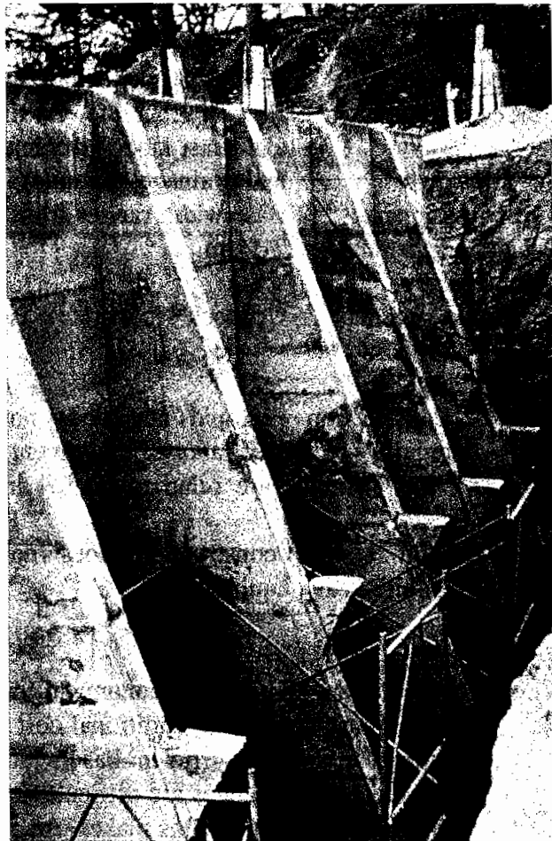
Counterfort wall prior to backfilling
