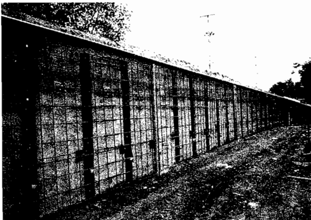
Soil-nailed wall before construction of permanent facing
