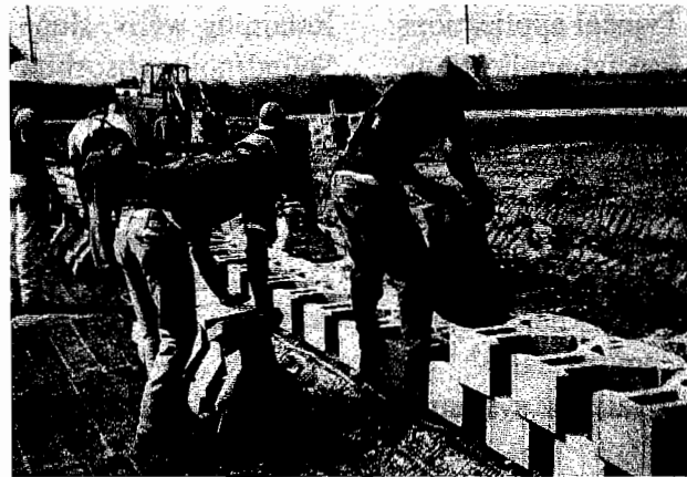
Construction of modular block wall
