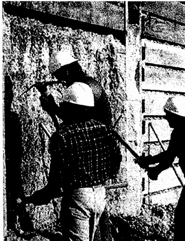
Figure 19. Installation of wood lagging.
