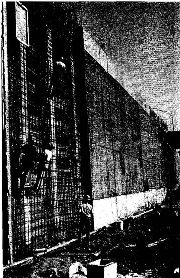
Figure 36. CIP permanent facing being constructed on an anchored wall.
