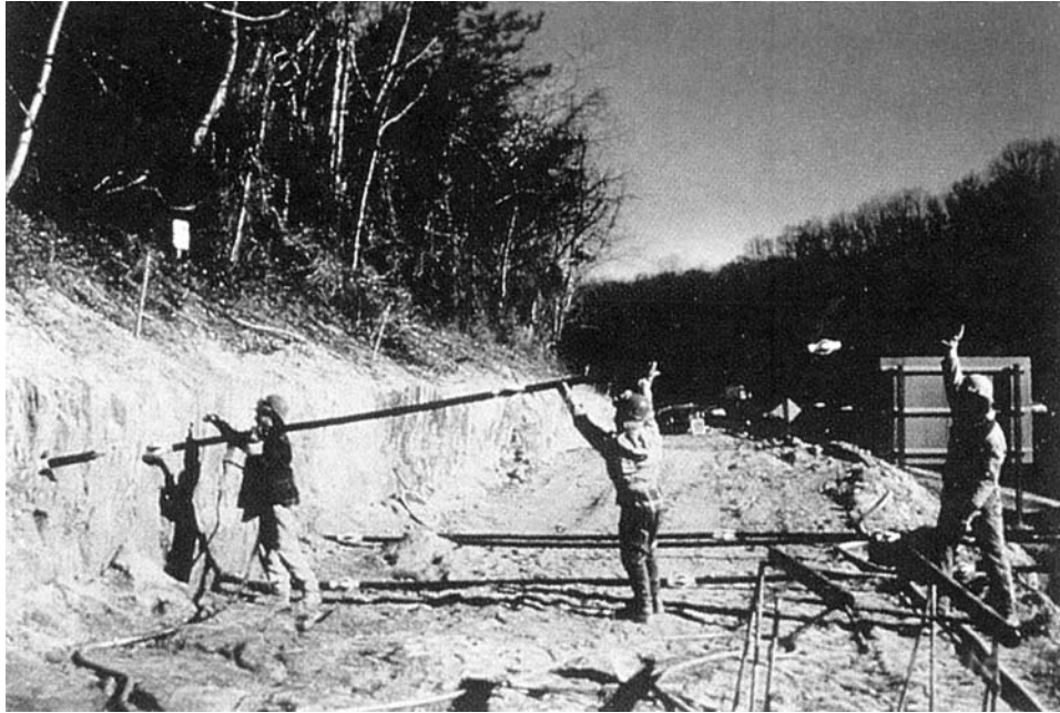
Figure 4.6: Initial Excavation Lift and Nail Installation.
