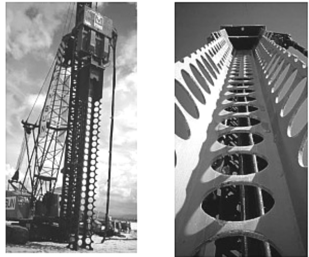
a) MRC compaction equipment b) MRC compaction probe
