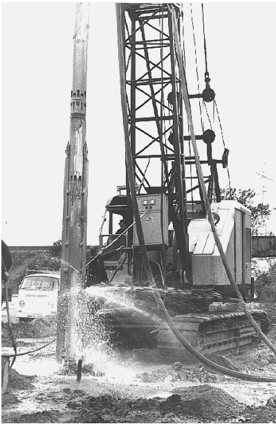
Figure 5. Vibroflotation equipment with water jetting
