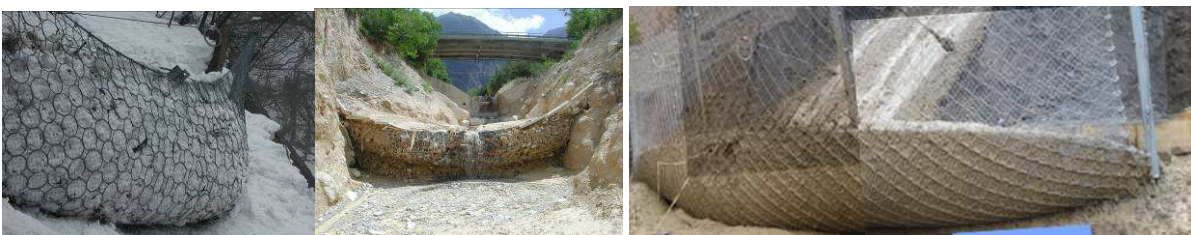
Fig. 6: Further usage of flexible protection measures against snow loads, debris flows or rockfall.
