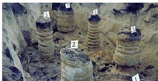
Figura 2: Columnas jet. Earth Tech Geotechnical Construction Services
