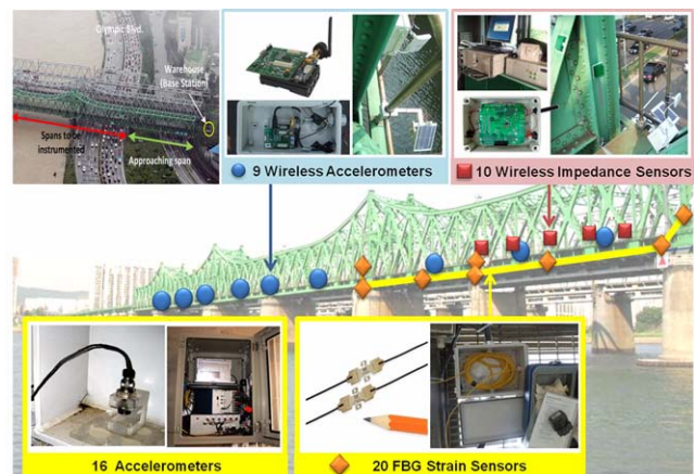
Fig. 15. SHM System on Han River Railroad Bridge
