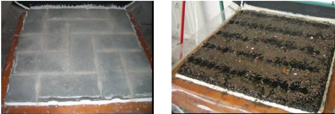
Figure 4. Pervious pavements of concrete blocks and porous asphalt completely clogged.
