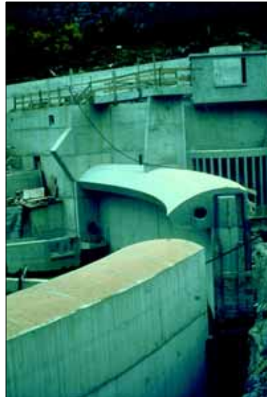
22 - Single curvature arch dam (Chapeauroux water intake). Note the standard crest shape of the overflow portion. (text p.115). ▶
