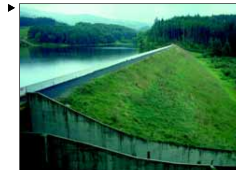
14 - Seeded downstream slope. (text p. 76-77).
