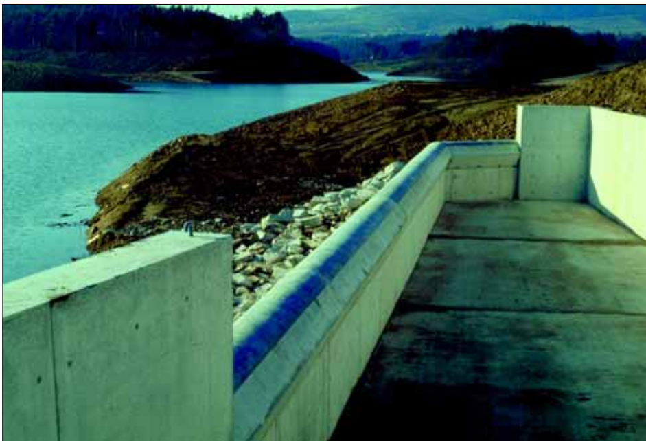
▼ 20 - Overspill part of a side inlet spillway.
