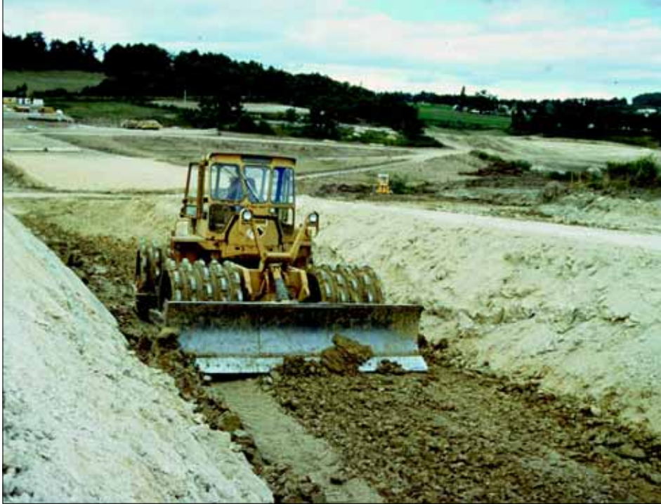
▲ 1 - Compacting clay in the cut-off trench (text p. 71).
