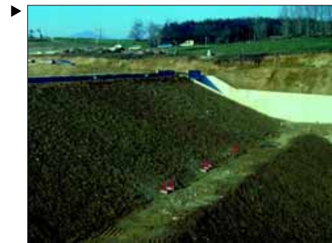
13 - Topsoil covering the downstream face of the same dam. Note the berm. (text p. 76).
