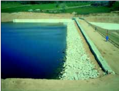
13 - Topsoil covering the downstream face of the same dam. Note the berm. (text p. 76).
