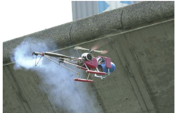
Fig. 4. Photo taken front the feasibility test done on the viaduct of Saint Cloud.
