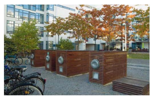
*Fig. 3.10. Collection points of the AVAC system fully integrated in the urban environment of Hammarby Sjöstad (source: Envacgroup).*
