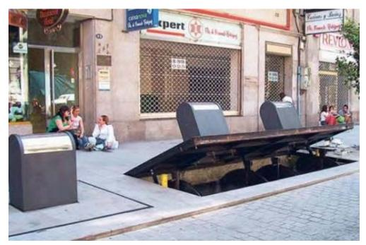
Fig. 3.7. Underground waste collection system operated in Adu Dhabi.
