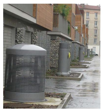
Fig. 3.9. View of the inlet points positioned outside the apartment buildings in Romainville.
