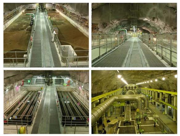
*Fig.* 2.11. Inside views of the rock caverns and the process installations in the Stanley underground *STP* (Hong Kong).
