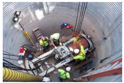
Fig. 3.3. Microtunelling operation for the construction of underground pipe AVAC infrastructure.
