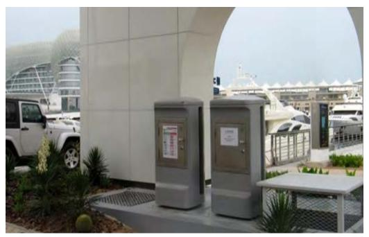
Fig. 3.6. Inlet points for the AVAC system in the Yas Island.
