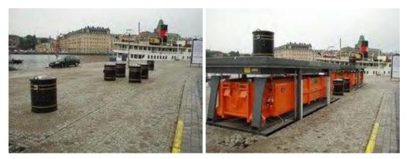
Fig. 2.6. Hydraulic underground compactor in normal and emptying position.
