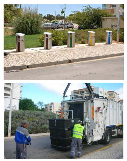
*Fig. 3.11. (a) Underground waste containers in Portimao (b) Waste collection process of the containers using specially adapted trucks.*
