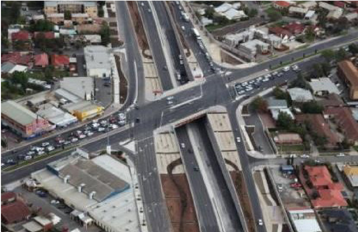
Illustration 4.9 - The completed gallipoli underpass
