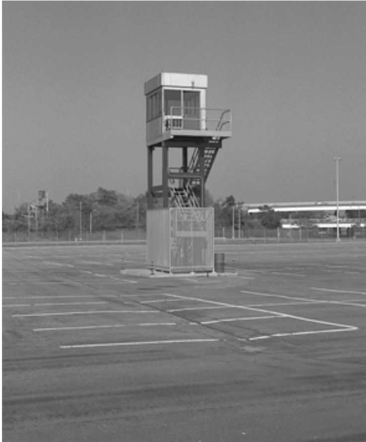
Designing a Defensible Space: On-Site Security Toweræ Howard Beach Park-and-Ride, New York City Transit, Queens, New York
