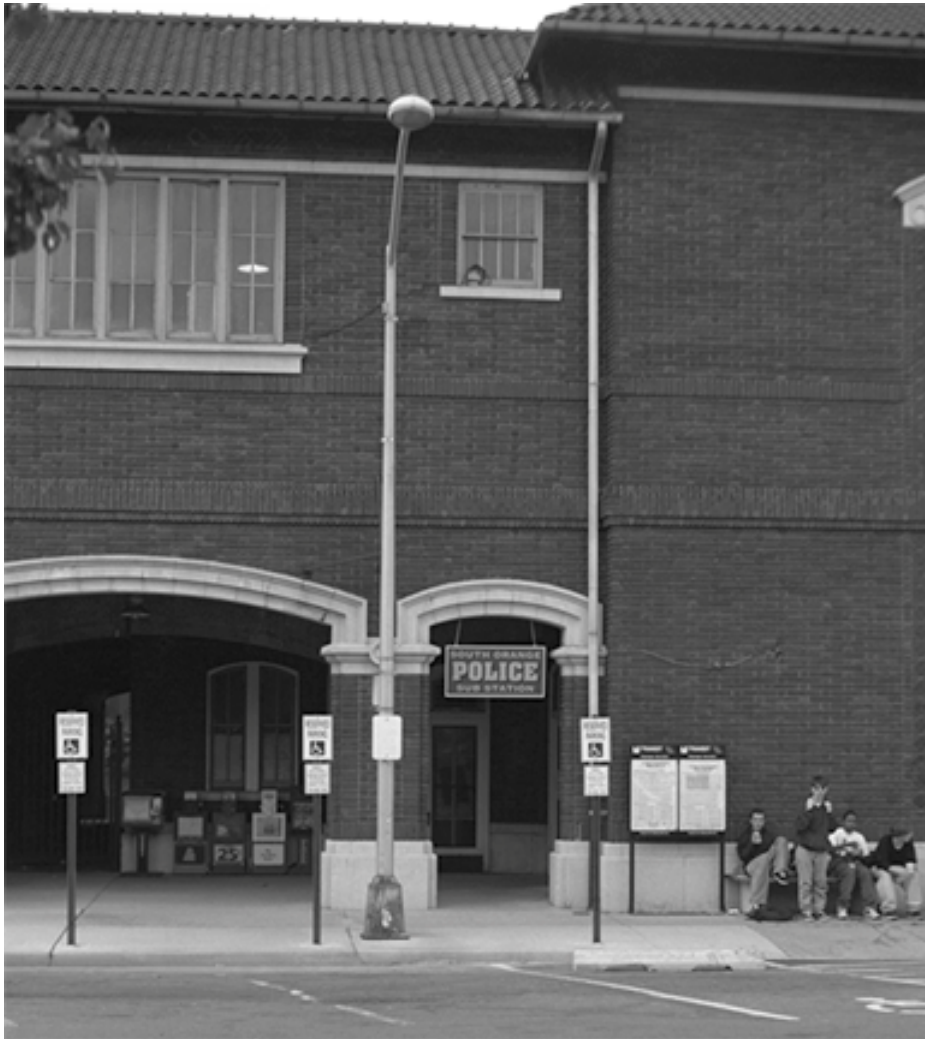
Joint Use Park-and-Ride FacilityæPolice Precinct in Transit Station South Orange Rail Station Park-and-Ride, NJ Transit, South Orange, New Jersey
