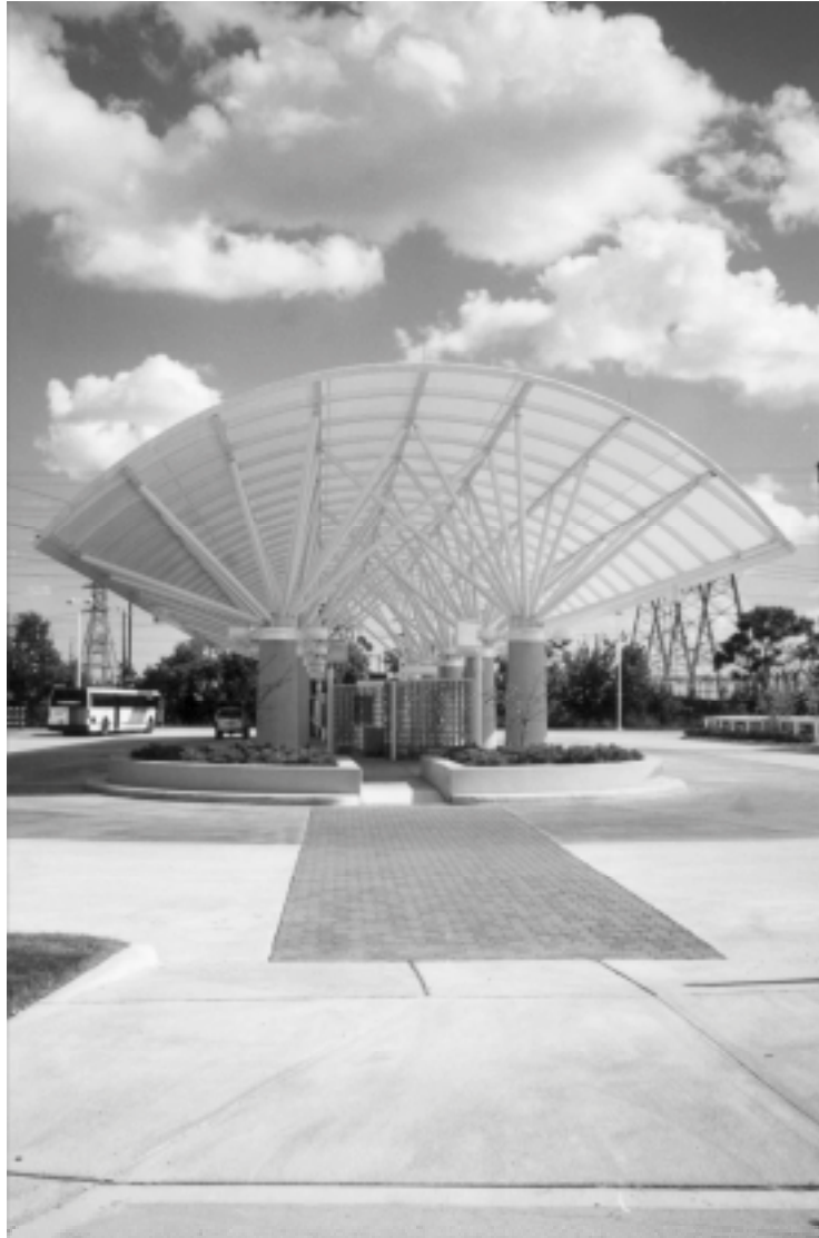
High Canopy Shelter Design to Allow for Air Flow in Hot Climate Gessner Park-and-Ride, Houston METRO, Houston, Texas
