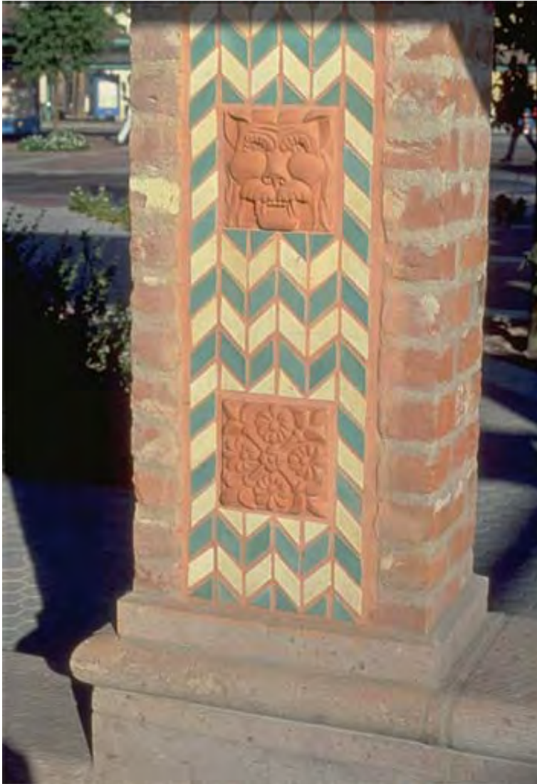
Tile WorkæTohno Tadi Transit Center and Park-and-Ride, Tucson, Arizona Photo Courtesy of City of Tucson
