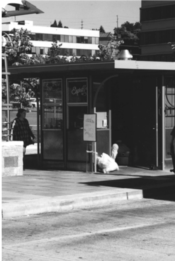
Joint Use Park-and-Ride Facility&Espresso Shop Northgate Transit Center and Park-and-Ride Facility
