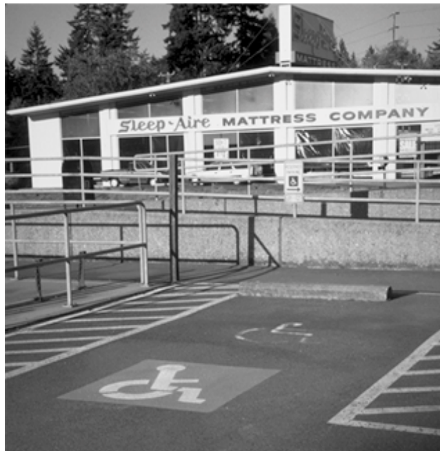
Designing a Defensible Space: Store Front Facing Park-and-Ride Facilityæ Shoreline Park-and-Ride, King County Department of Transportation, Shoreline, Washington
