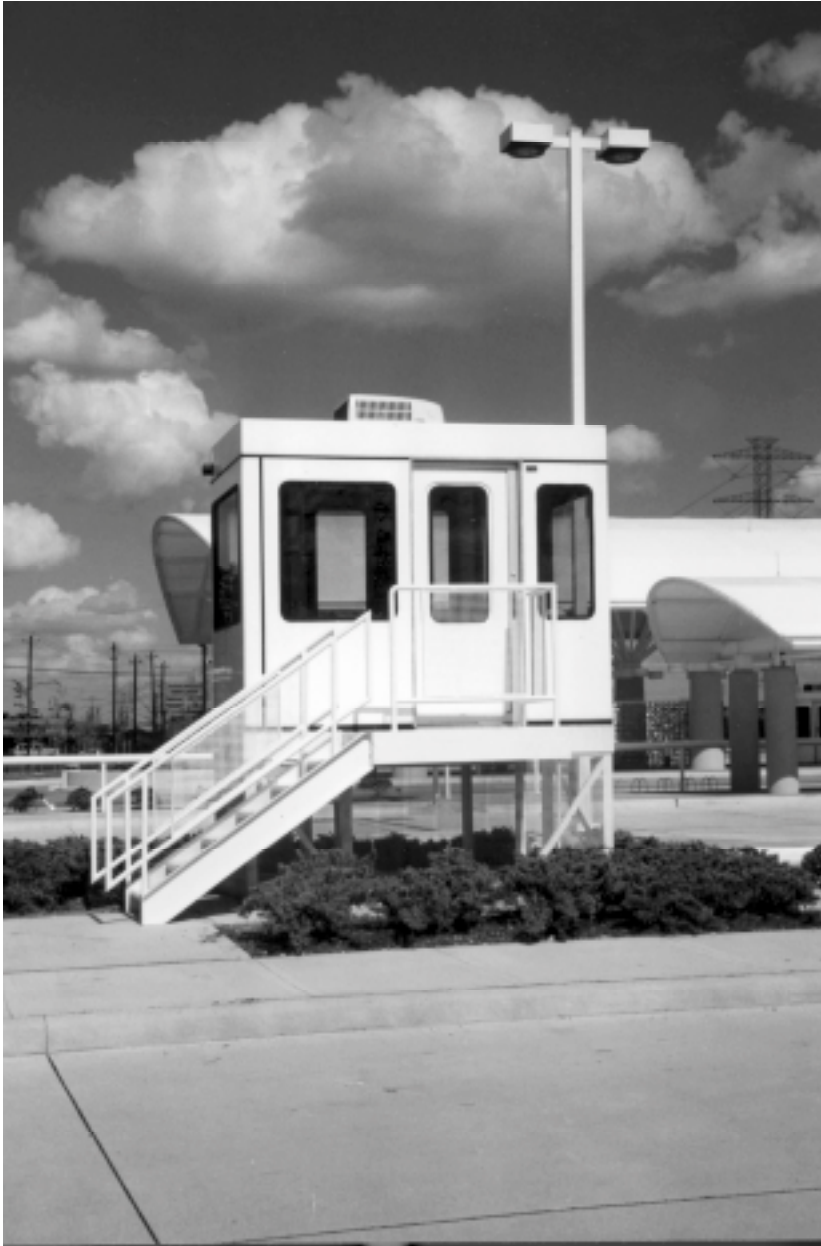
Designing a Defensible Space: On-Site Security Parking Attendant Officeæ Gessner Park-and-Ride, Houston METRO, Houston, Texas
