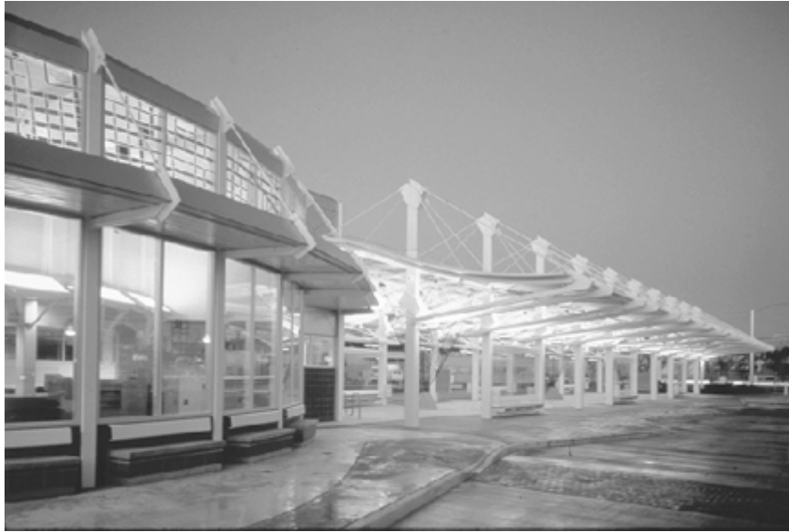
Enclosed Passenger Shelter to Protect Passengers in Colder Climate Olympia Transit Center, Olympia, Washington
