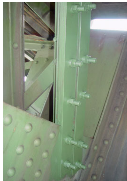
Fig. 8. Upgraded area within a strut
