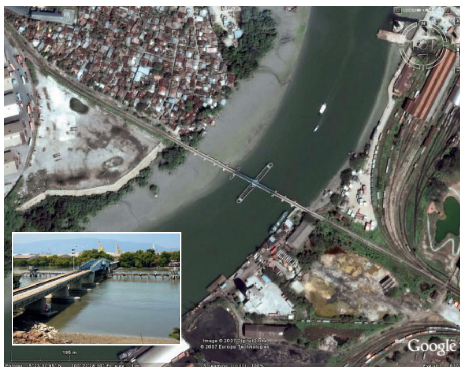
Fig. 1. Existing river bridge
